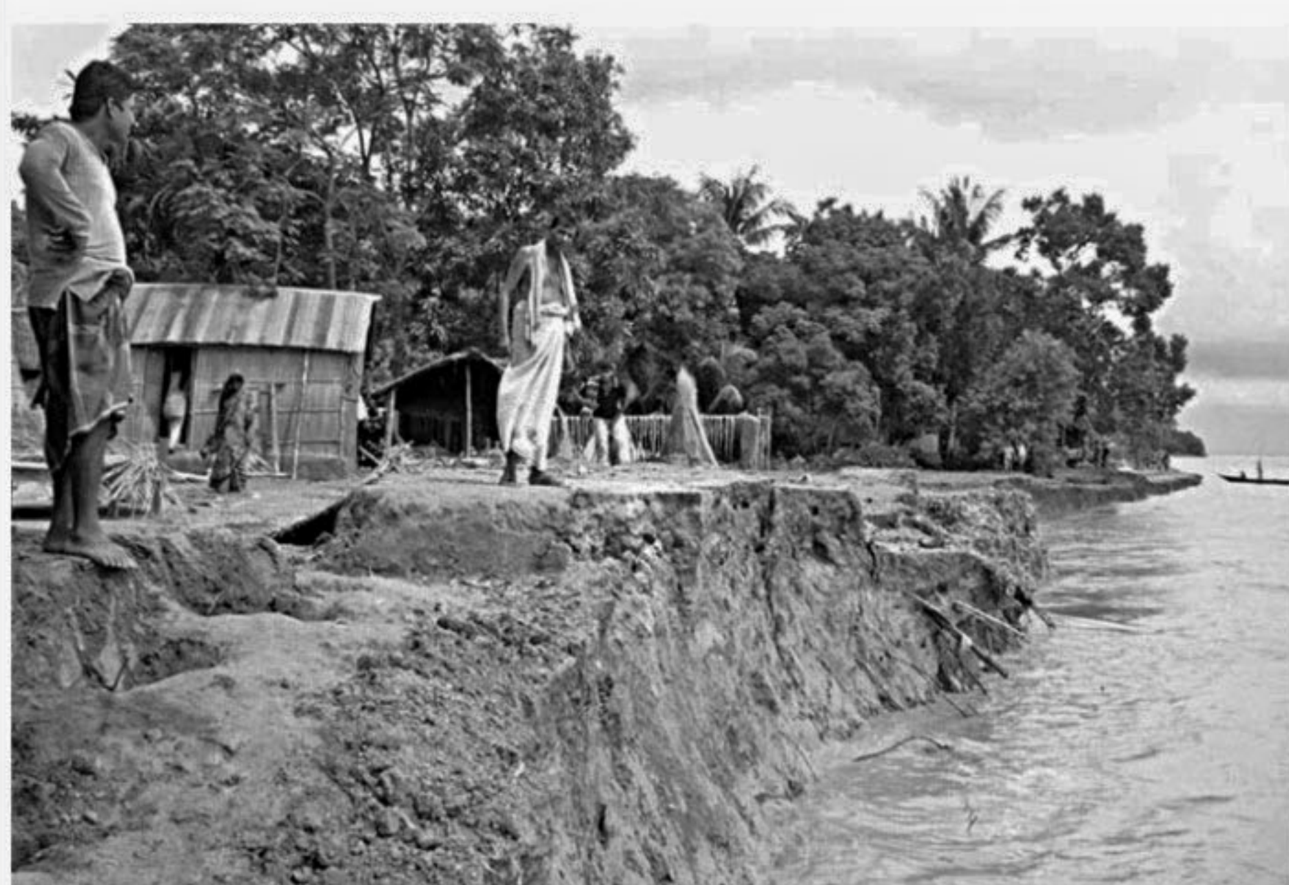
Erosion by the Padma has taken a serious turn, devouring at least 18 houses at Naruhati and Singhanagar villages in Satbaria union of Sujanagar upazila in Pabna district in a week.
