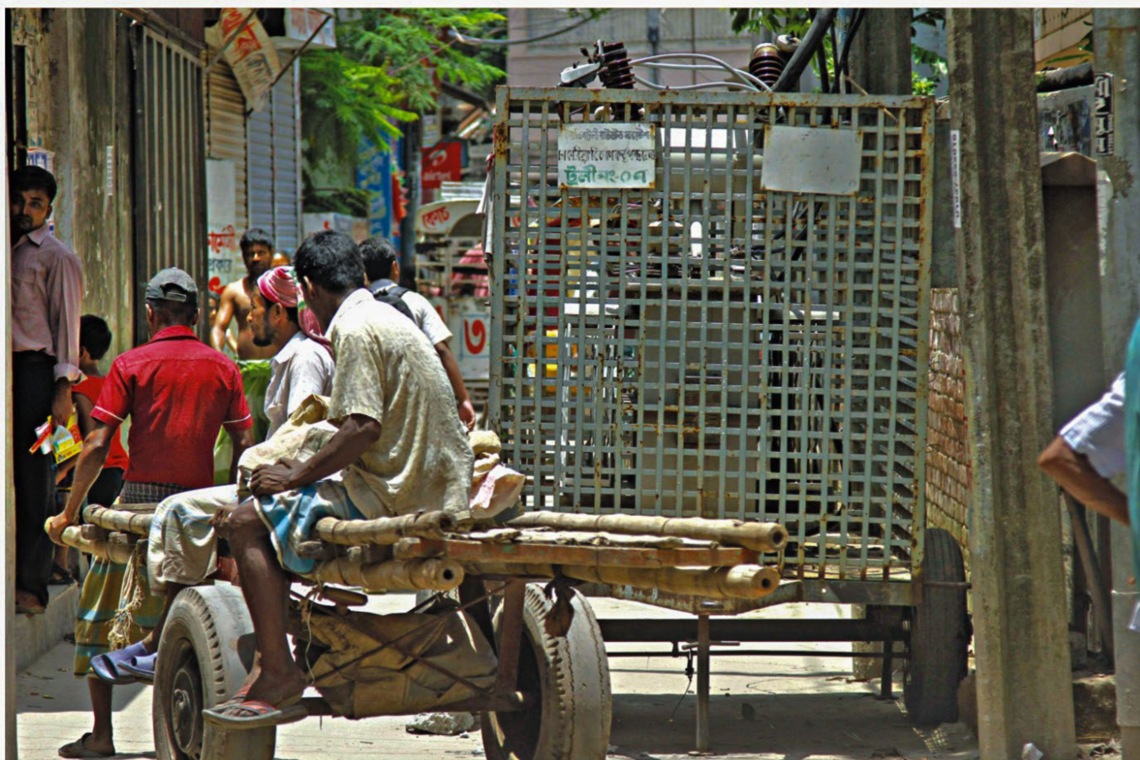
This photo snapped yesterday shows that an electric transformer has been set up in the middle of the road instead of electric pole at Uttar Mugdapara in the city creating obstacles to movement of vehicles as well as commuters.
