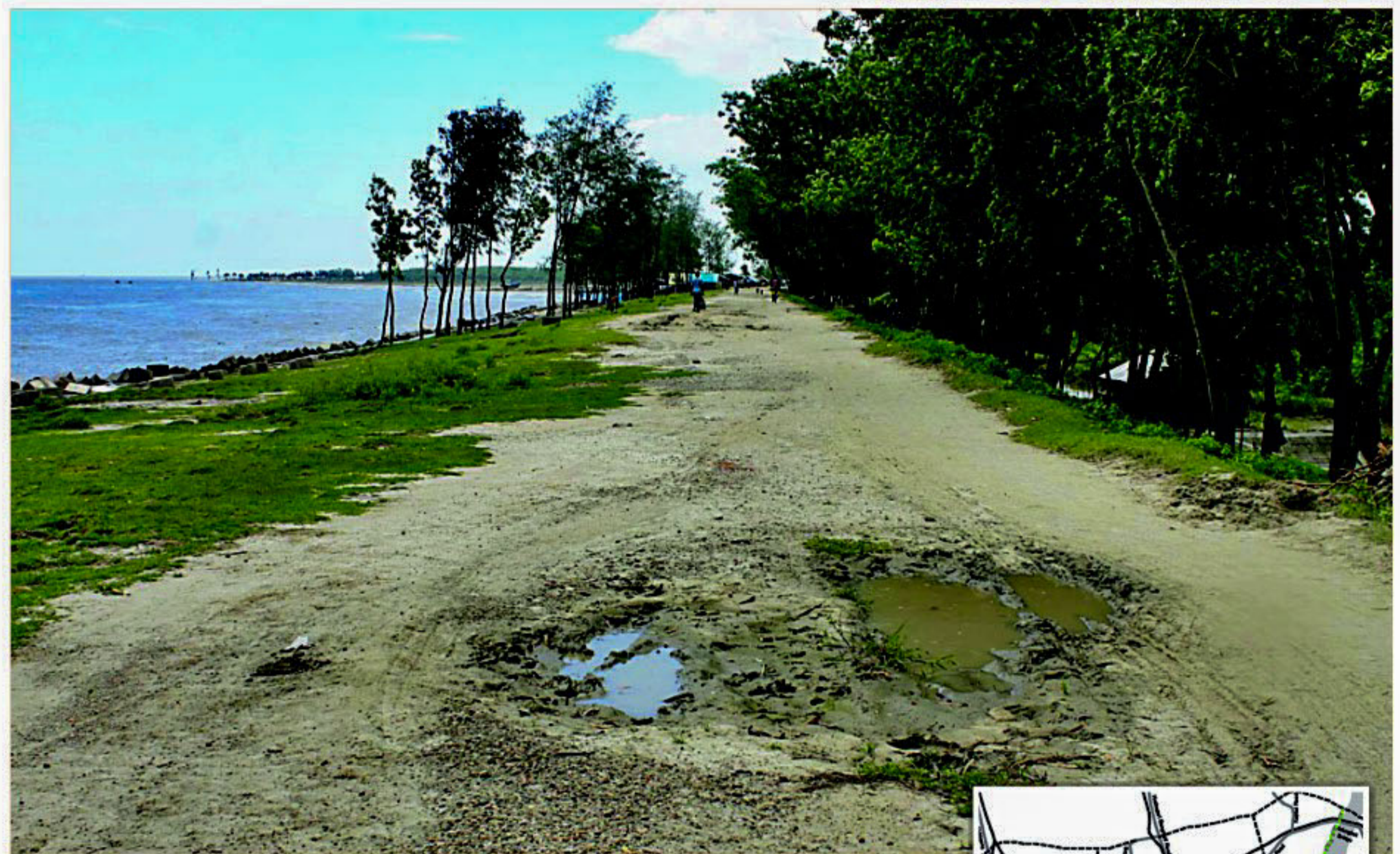
Outer Ring Road on the embankment along the Bay of Bengal.
