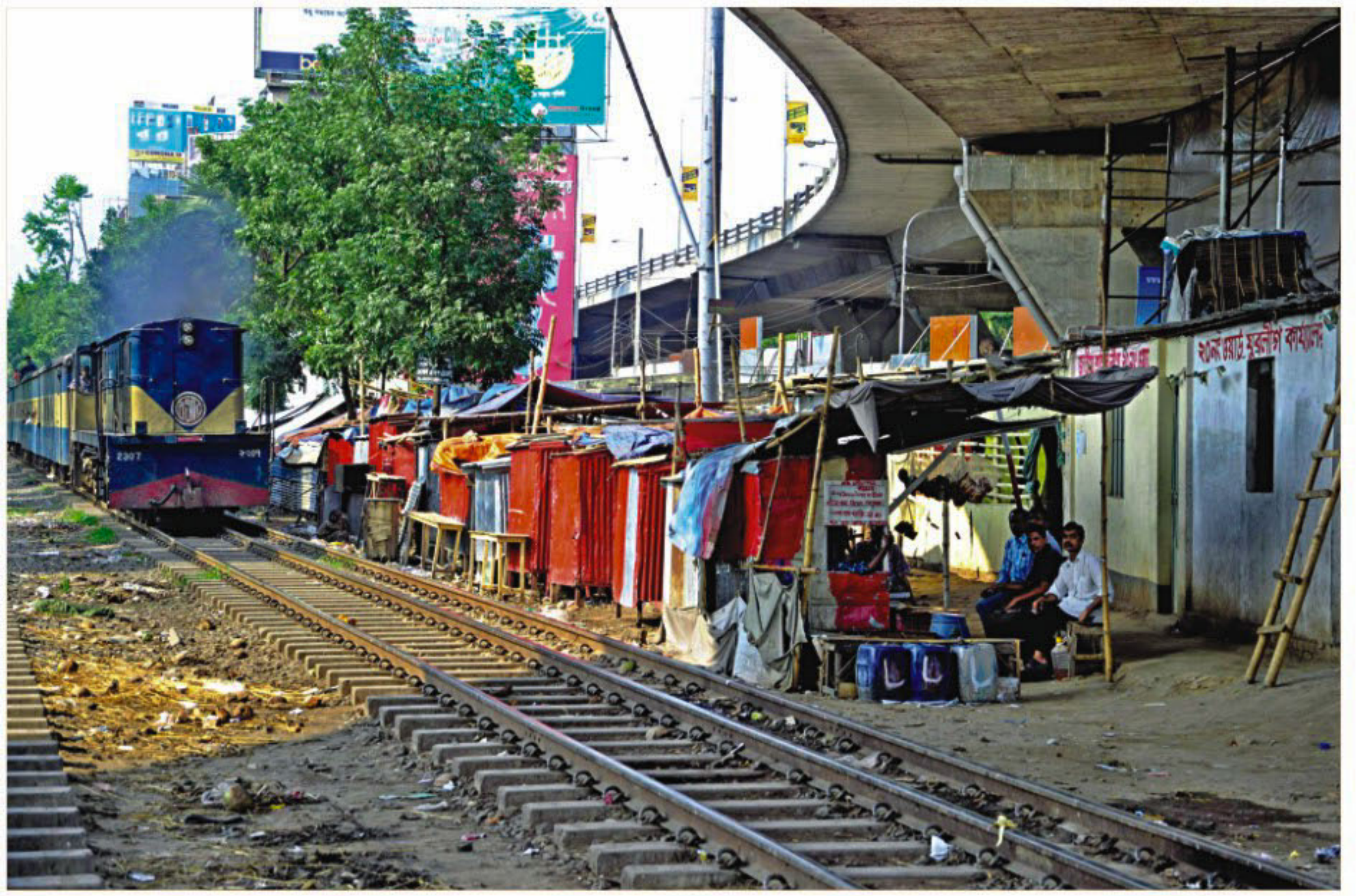
Tea stalls and other illegal structures are built perilously close to the rail lines under the Mohakhali flyover in the capital. The photo was taken yesterday.
