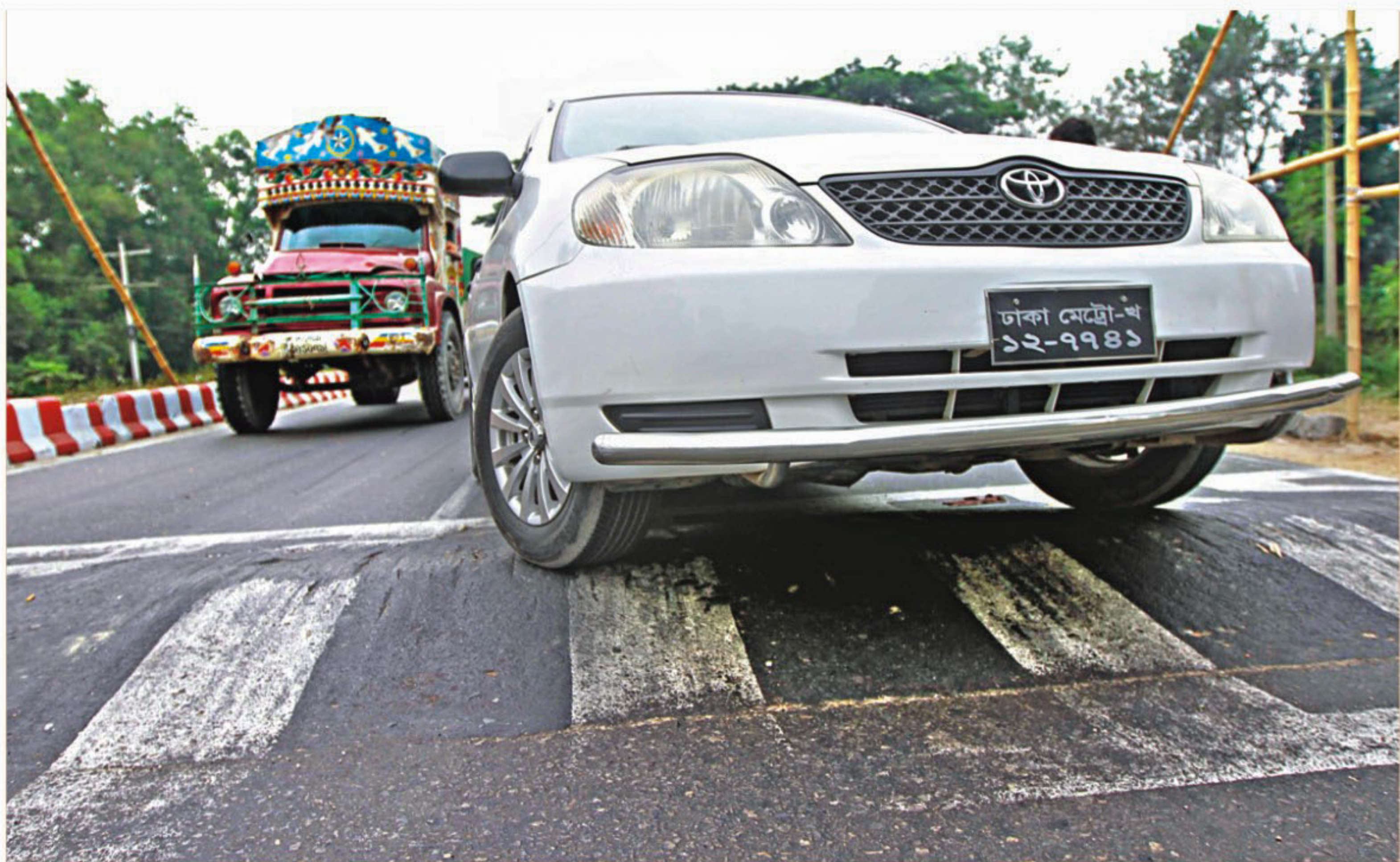
A car goes over a speed breaker in an angle so that it does not scrape its bottom on the high bump. A large number of the speed breakers in the country are too high for small vehicles to scale over comfortably even at crawling speed. The photo was taken near Jahangirnagar University on Dhaka-Paturia Highway.
