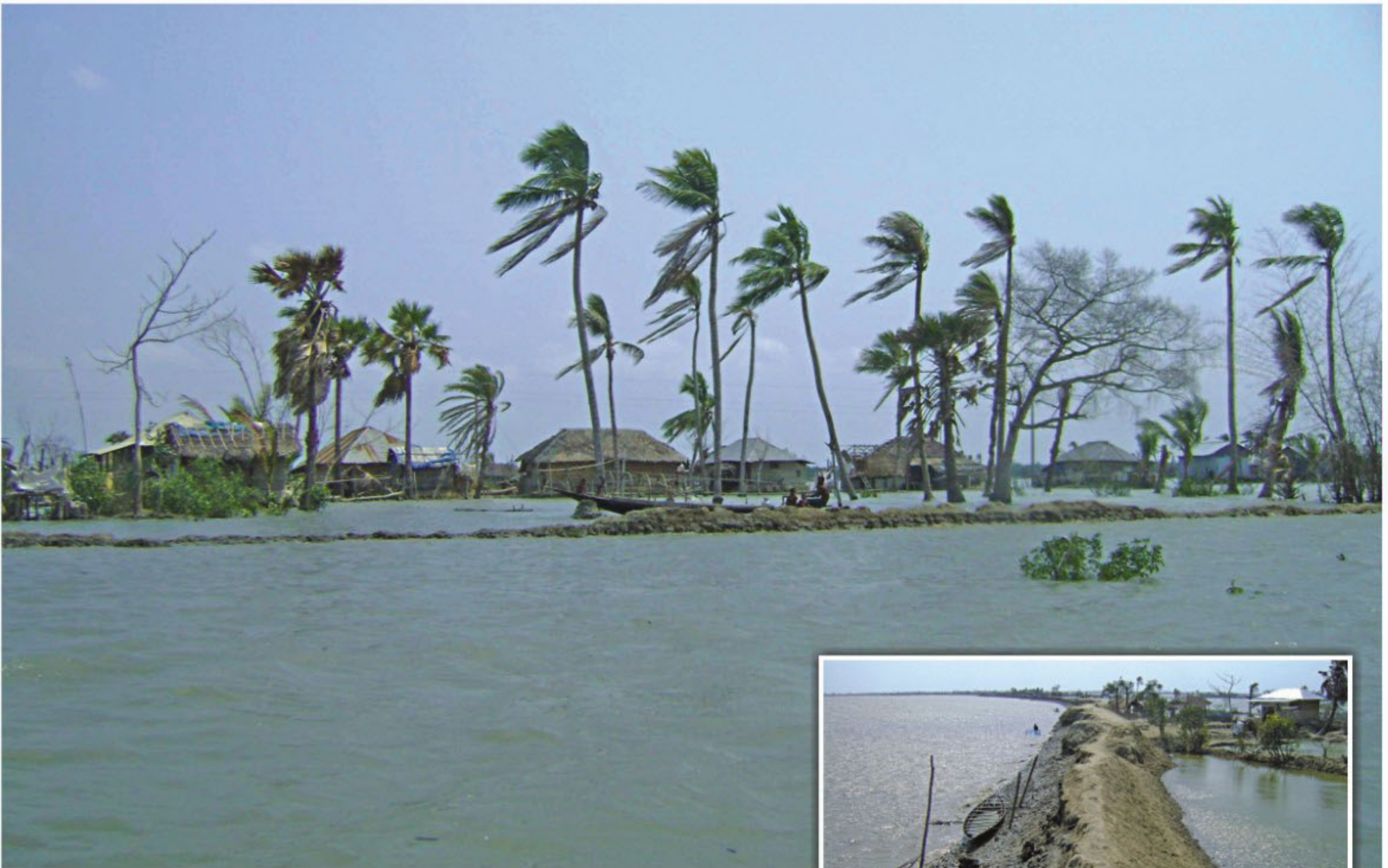
Twice a day during high tide the 5,000-acre land at Koira in Khulna is inundated by saline water rushing through the breach cyclone Aila had created in the coastal line embankment two years back. Inset, the coastal embankment that requires urgent repair.
