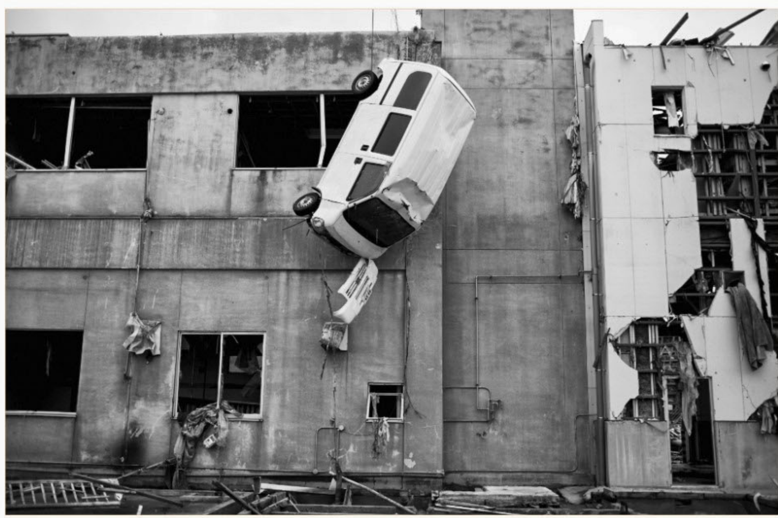
A car hangs from a damaged building in Onagawa town, Miyagi prefecture yesterday. The death toll from a massive earthquake and tsunami that devastated Japan's northeast coast topped 10,000, two weeks after the disaster struck, the National Police Agency said.
