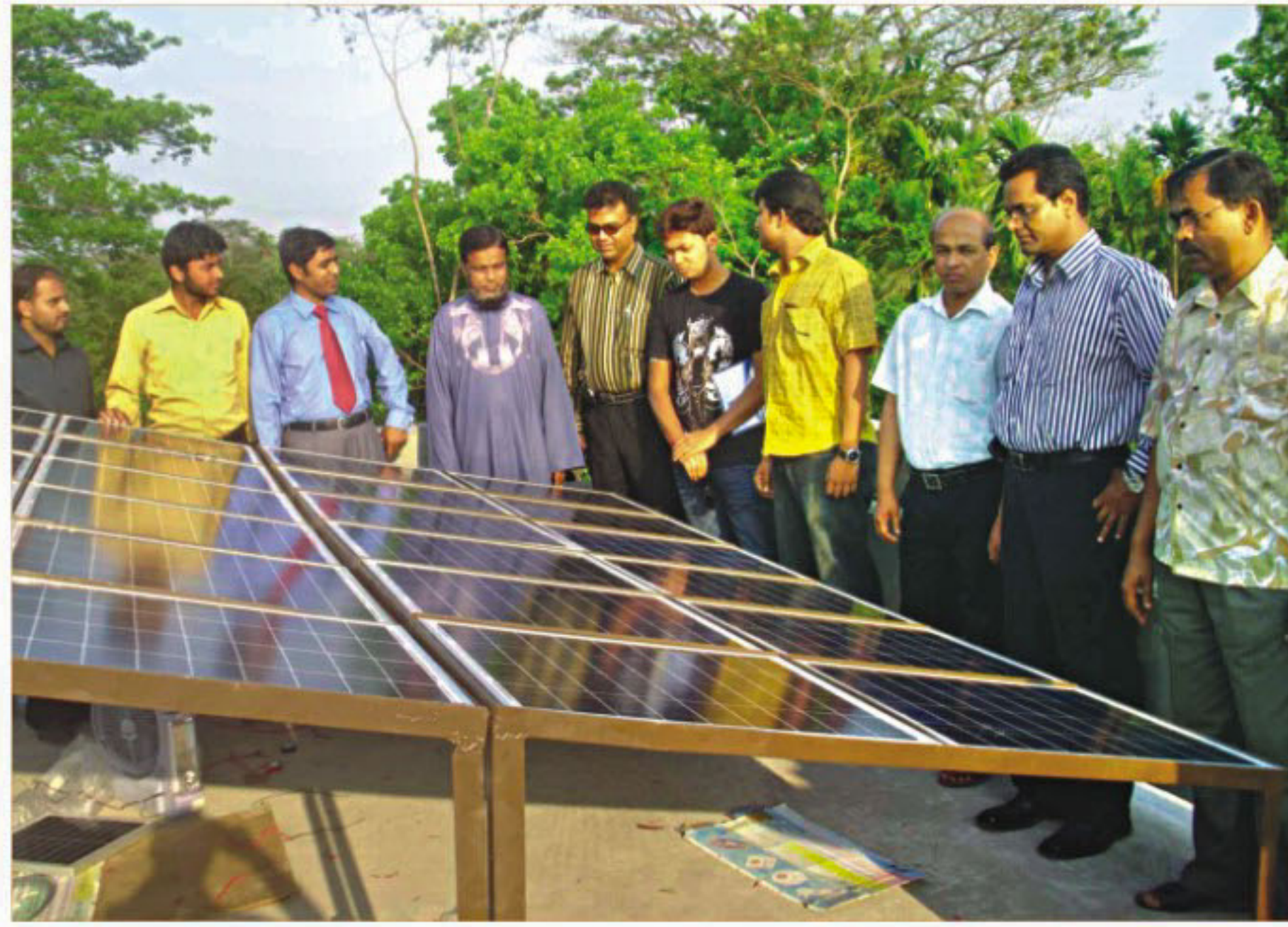
STAR Officials launch a solar power pilot project at a factory of Amrita Food Products in Barisal on Thursday. Bangladesh Solar Energy installed the 1,500 watt system.
