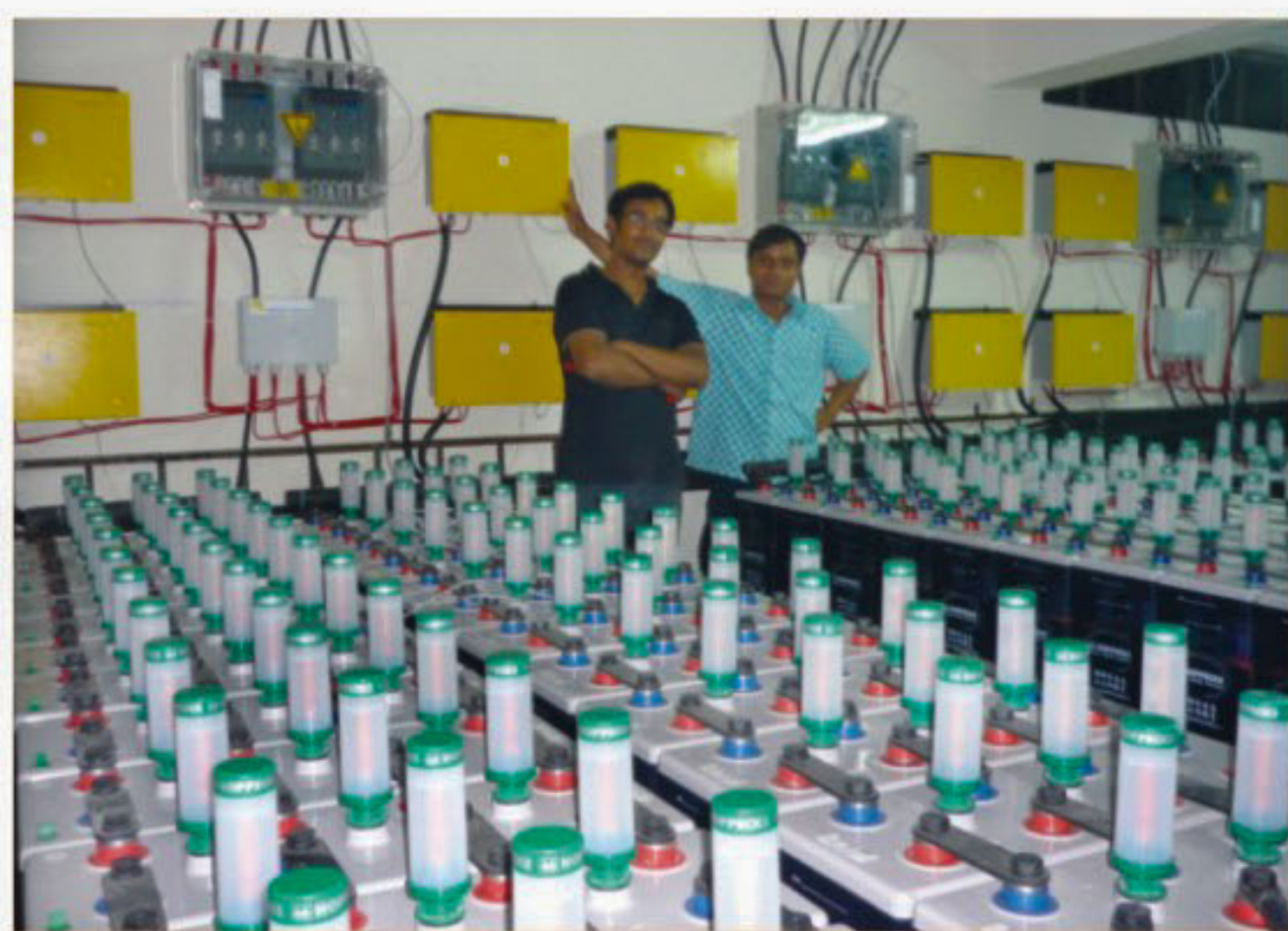
German batteries that store power from the solar panels.
