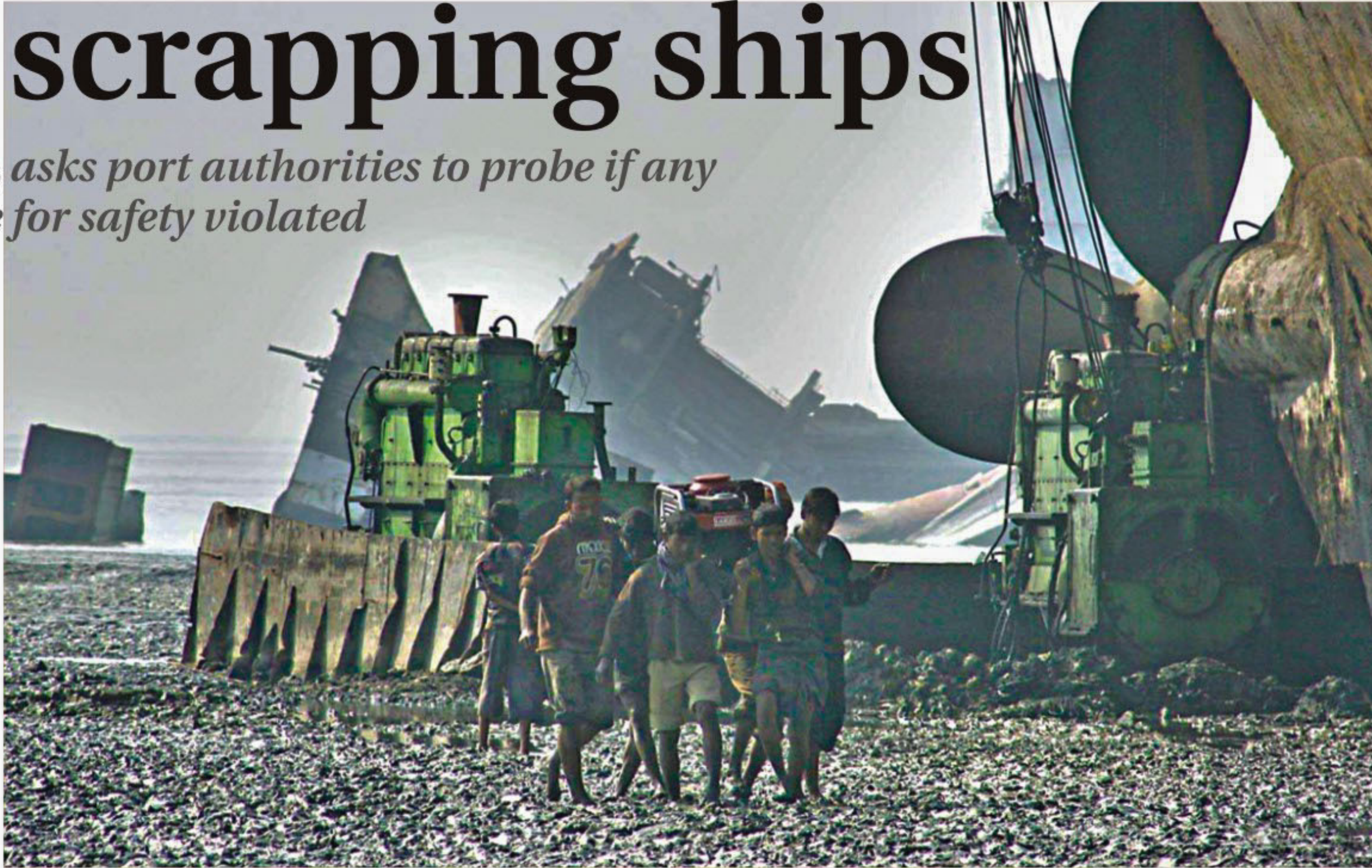
The campaign to ensure safety for workers at ship-breaking yards apparently had little impact. This photo taken in Chittagong yesterday shows workers doing the heavy lifting without even shoes.
