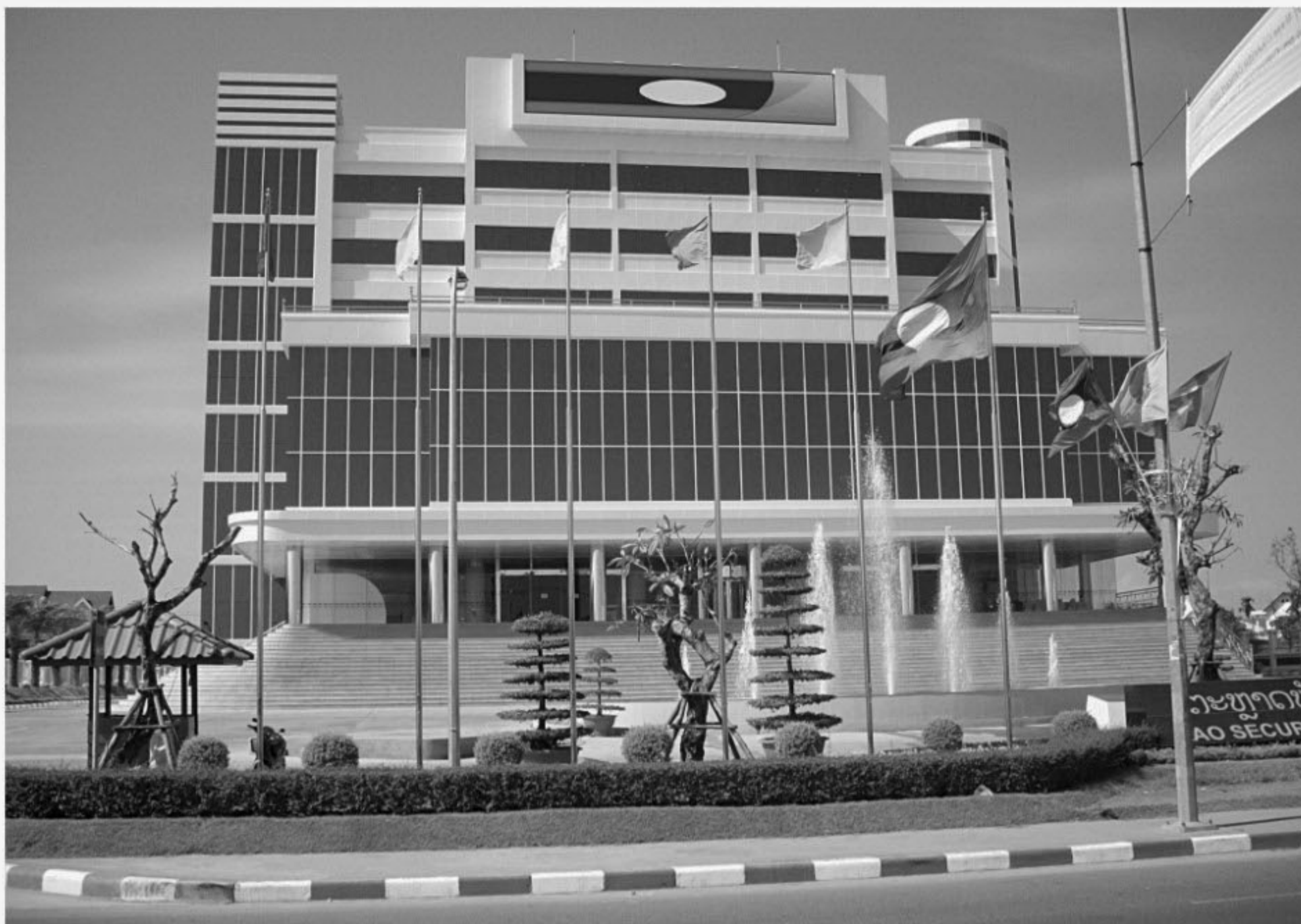
A view of the Laos stock exchange building in Vientiane. Laos opened its stockmarket, which is expected to pull in foreign investors.
