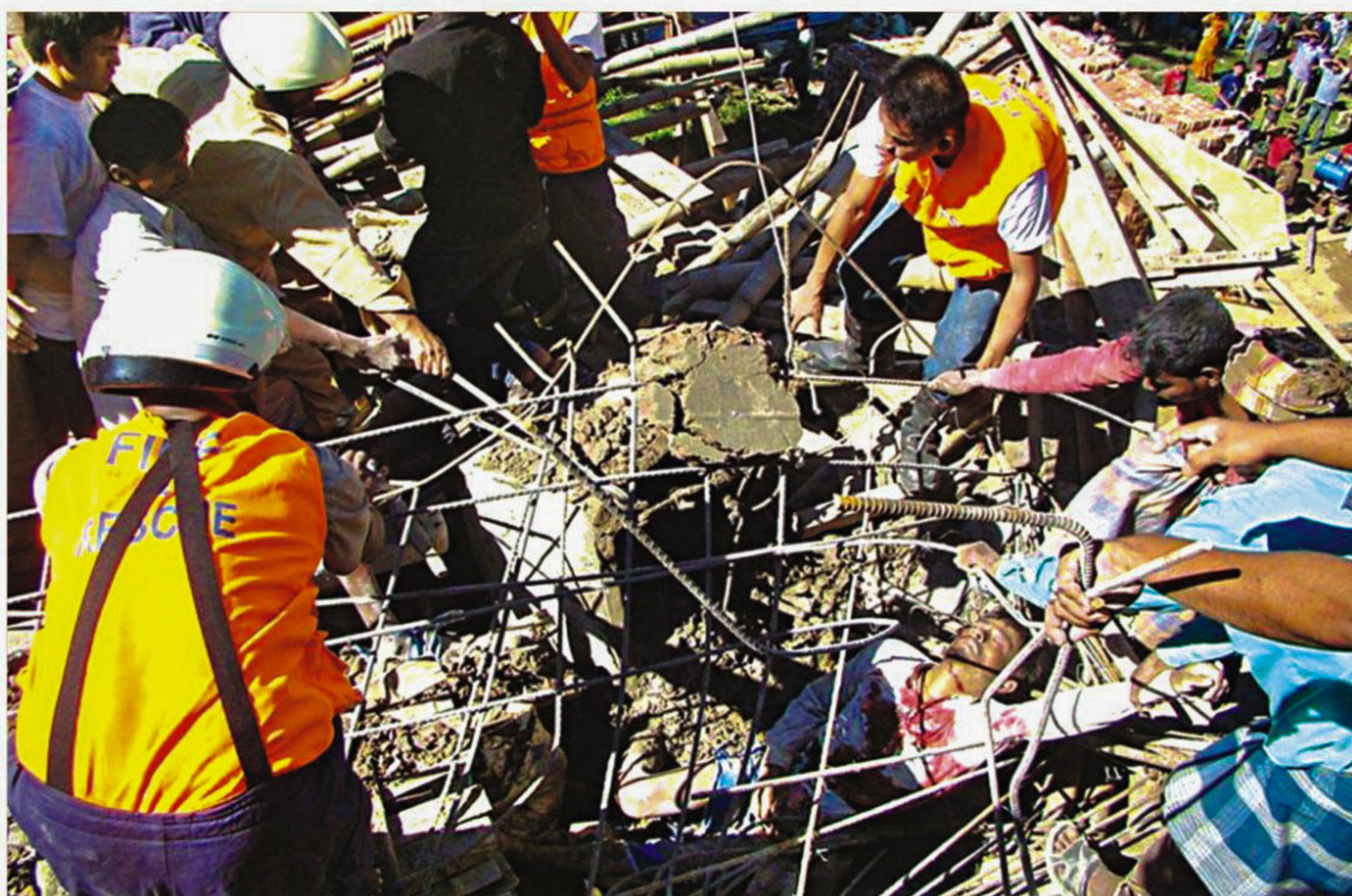
Rescuers try to get a worker out of the rubble after the roof of the under-construction Fatema Rani church in Bandarban collapsed killing a person.
