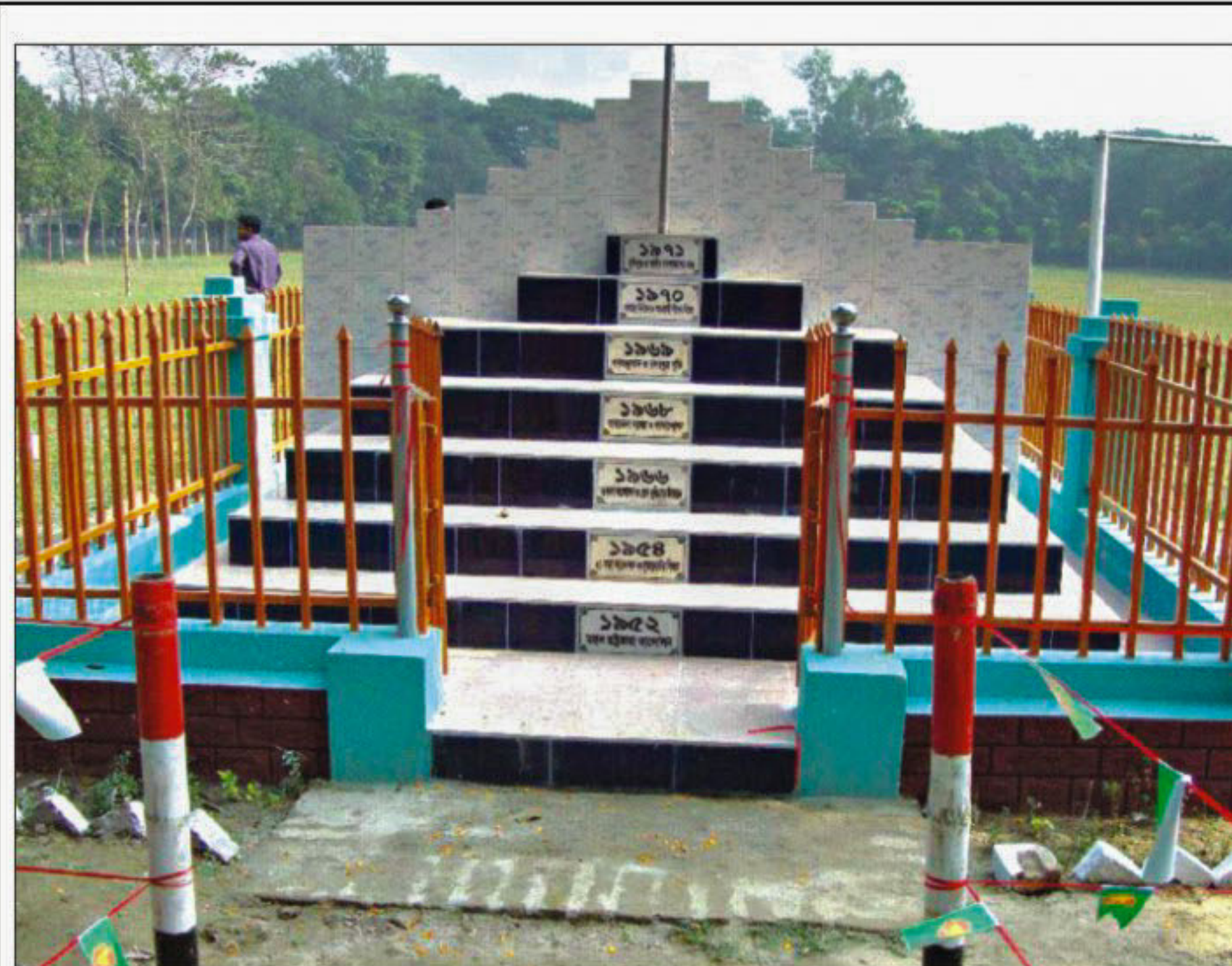
Swapno Siri, a monument designed in a set of steps to quickly recall our history of movement from 1952 to 1971, was inaugurated at Lalmonirhat Govt College premises yesterday.
