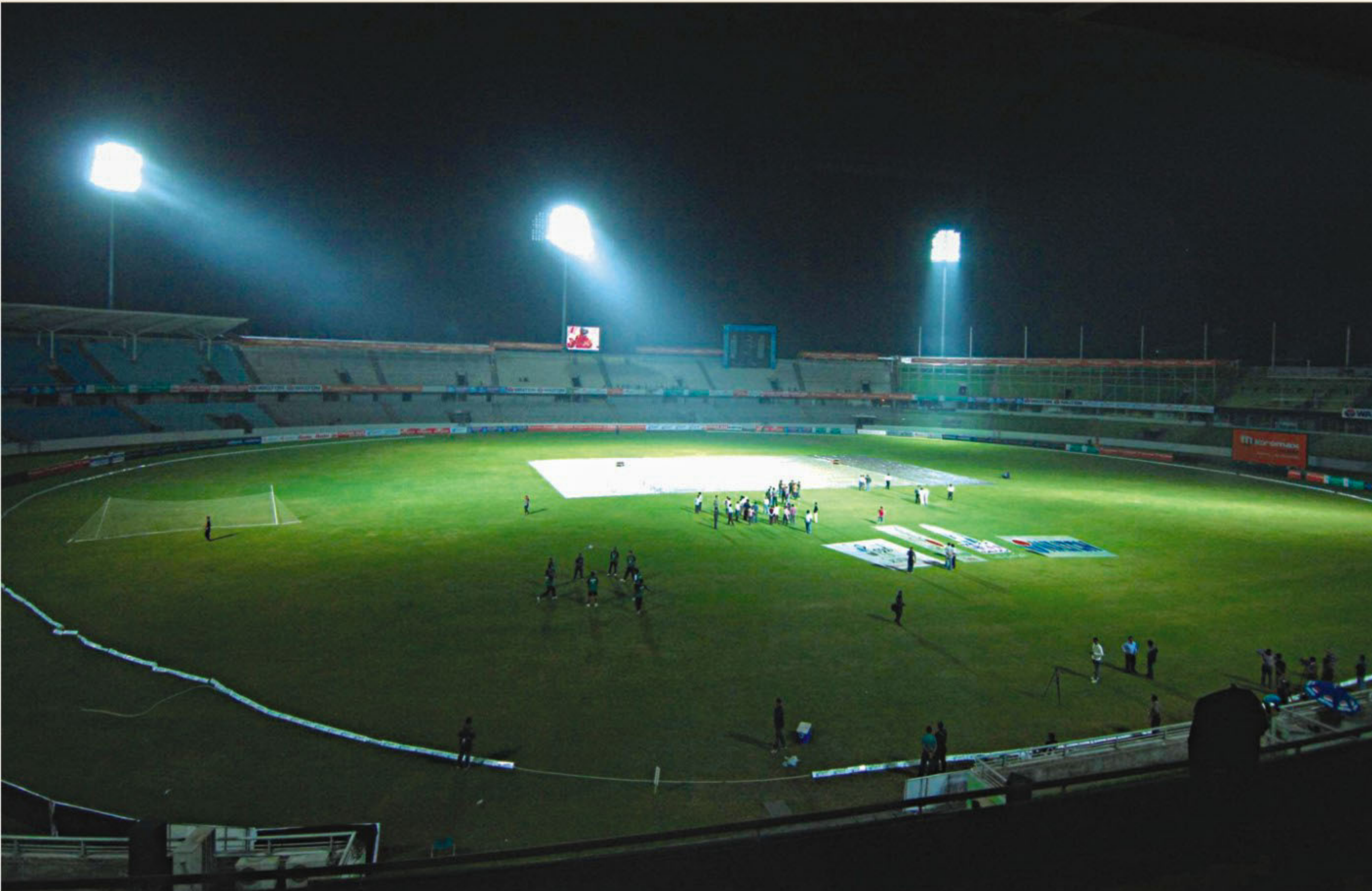
NOT QUITE READY: The test run of the new floodlights at the Sher-e-Bangla National Stadium on Sunday revealed that the focus of the lights was skewed towards the centre of the pitch, rather than on the entire field. As a result, today's day-night fixture between Bangladesh and Zimbabwe has been changed to a day affair.
