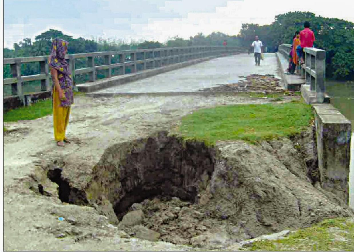
This bridge over Kumer River in Shailkupa upazila of Jhenidah district has remained virtually unusable even after three years of its construction due to lack of an approach road and wing walls.
