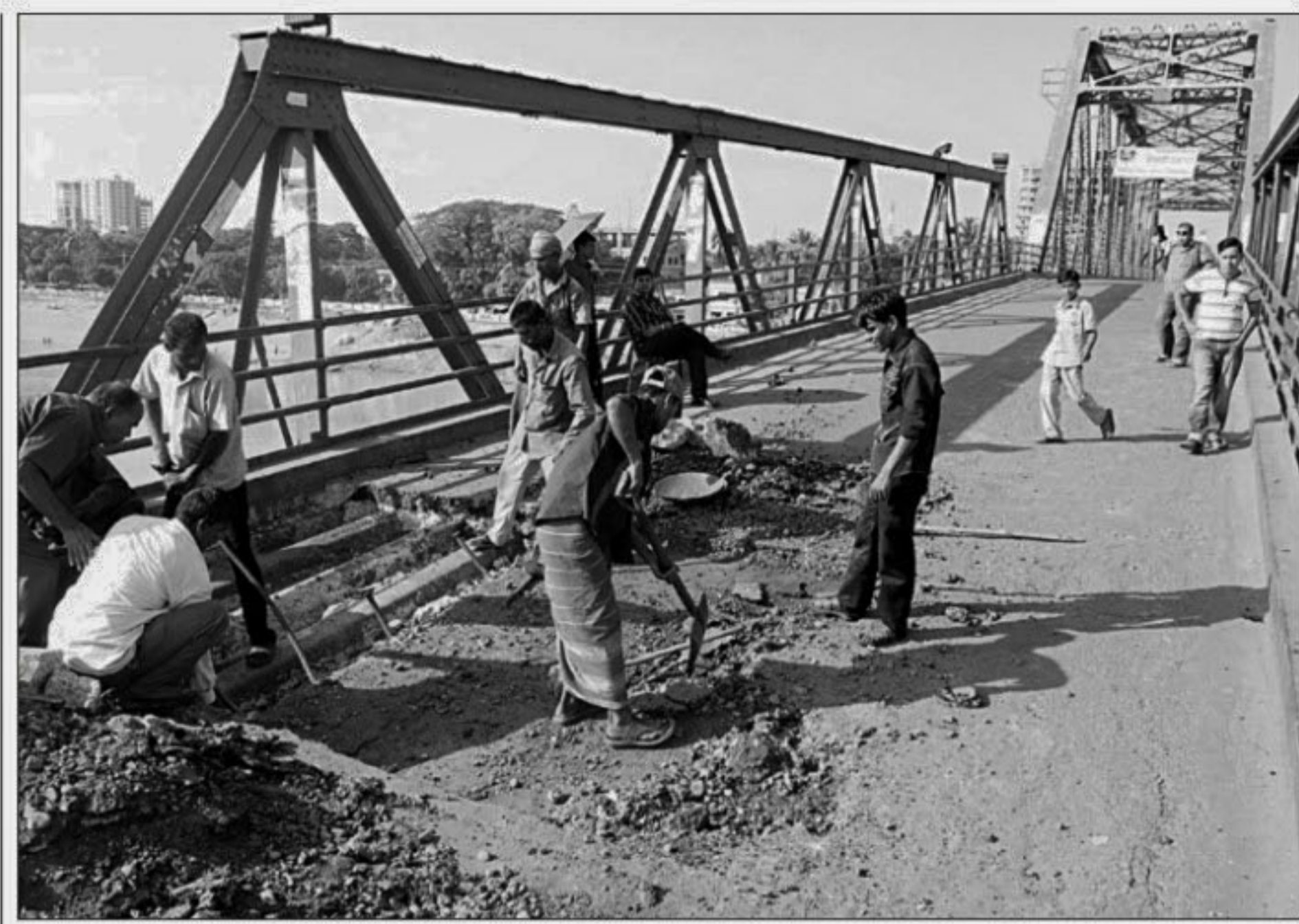
Workers of Roads and Highways Department doing repair work on Keane Bridge across the Surma River in Sylhet as a 10-foot-long plate collapsed yesterday due to unauthorised movement of heavy vehicles.
