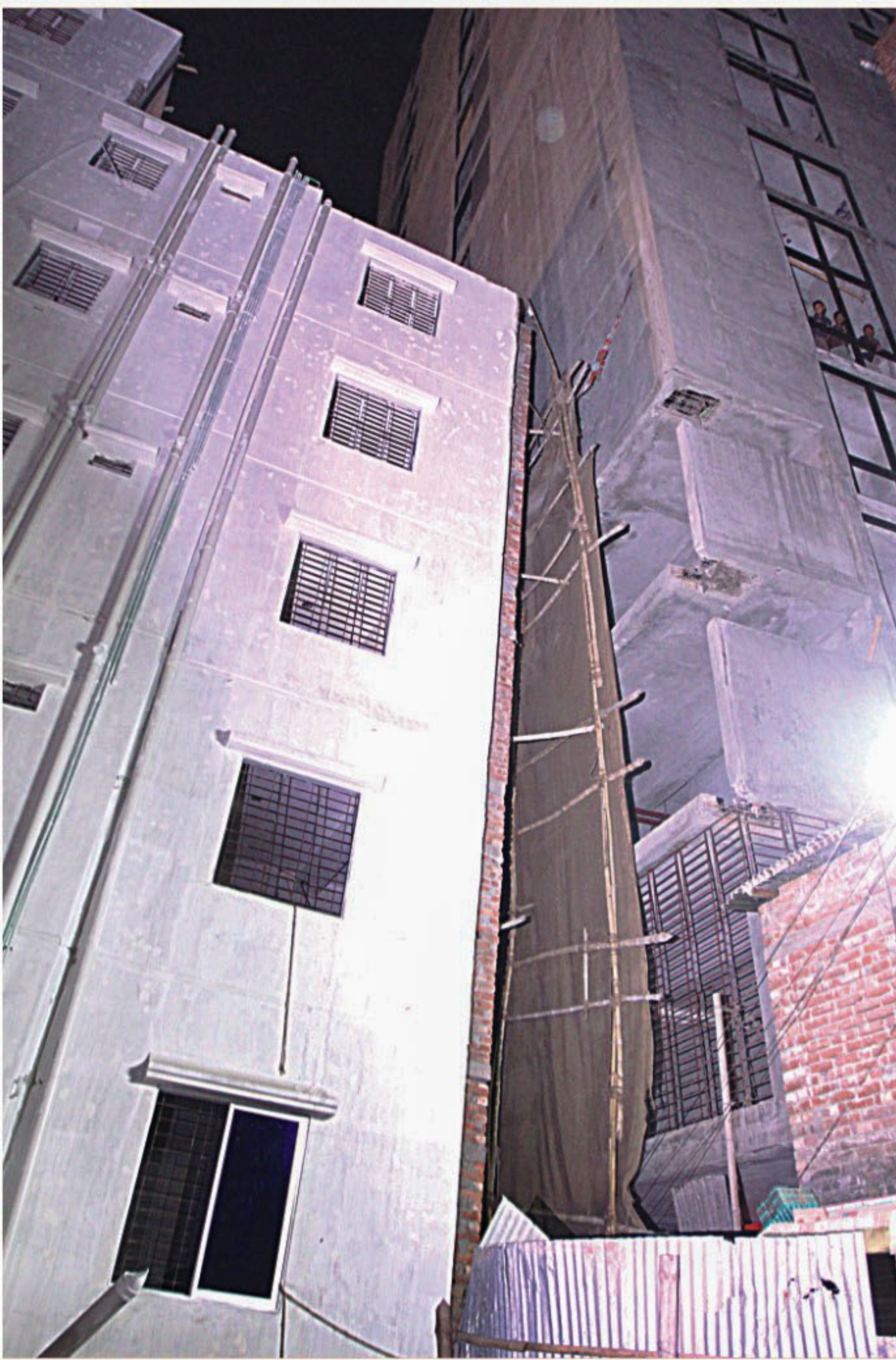
Domino effect takes place from a seven-storey building in Kanthalbagan, Dhaka after it tilts on an adjacent 17-storey building making the second one tips onto another 10-storey residential unit. The incident happened when a pillar in the basement of the seven-storey building collapsed last night.
