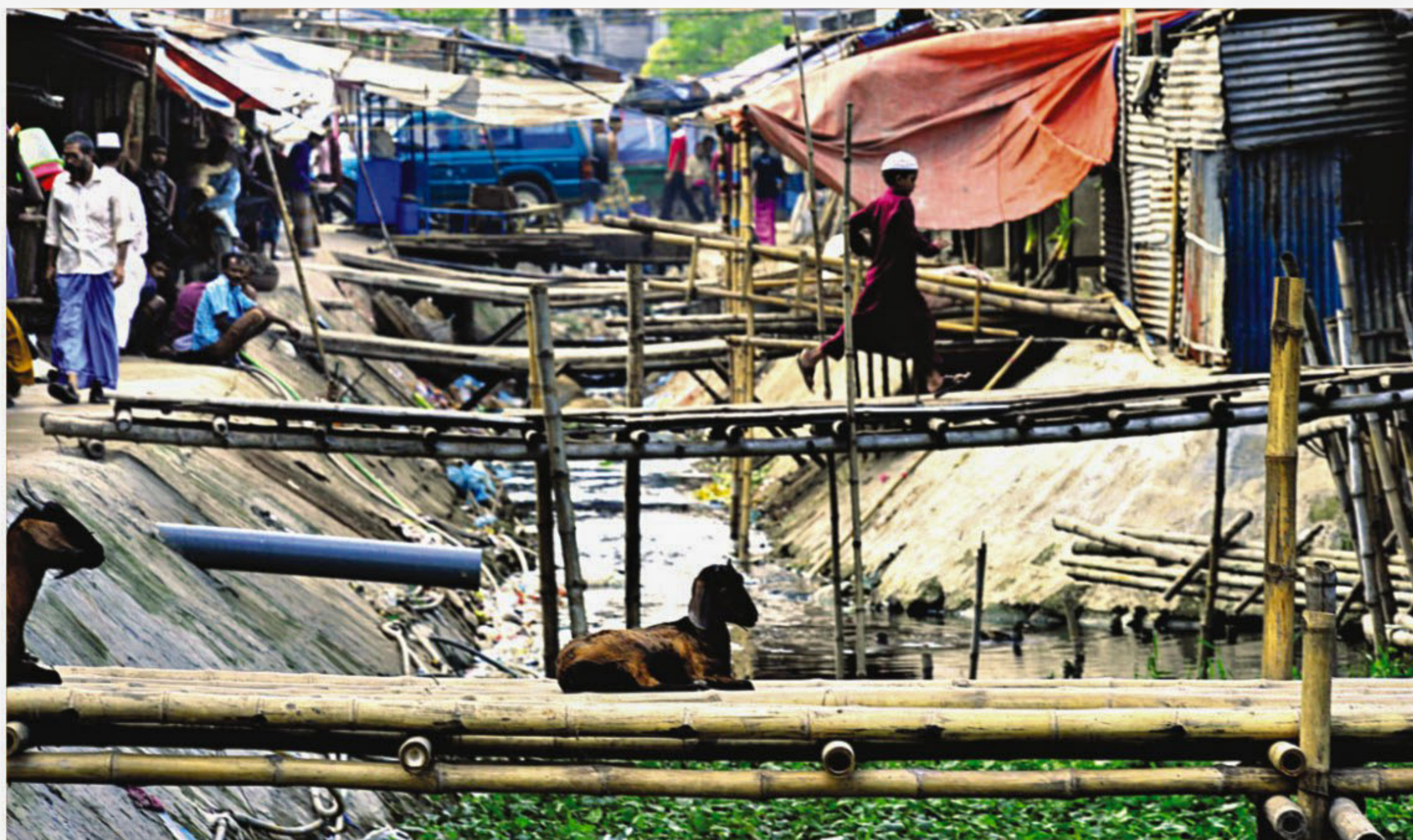
Dhaka Wasa removed illegal structures on the Kalyanpur Canal at Kazi Office Road-2 in Shyamoli earlier this year but as seen in most such cases, the banks have been encroached upon again. The photo was taken recently.
