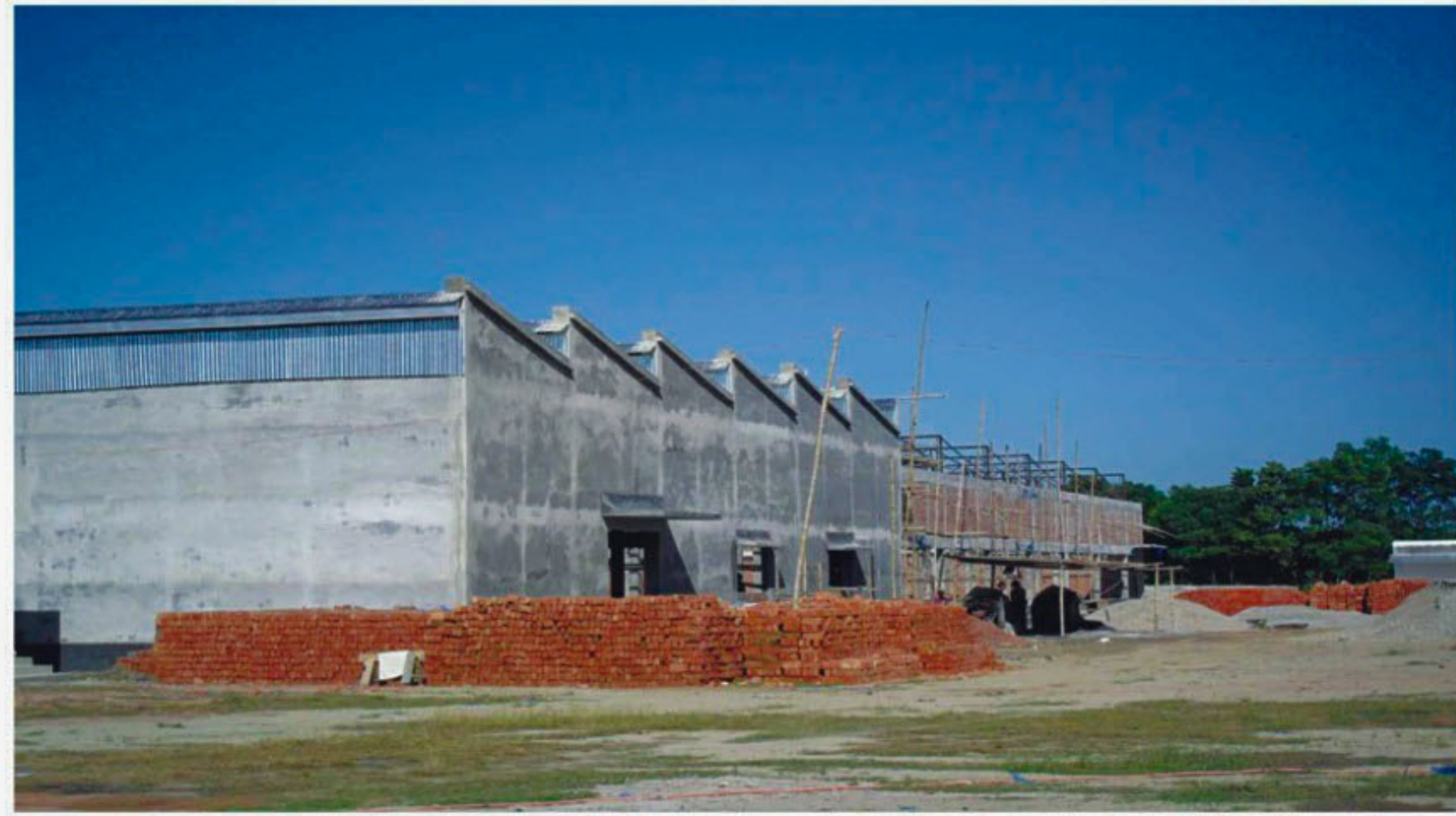
An under-construction building of Azad Jute Mills in Lalmonirhat.
