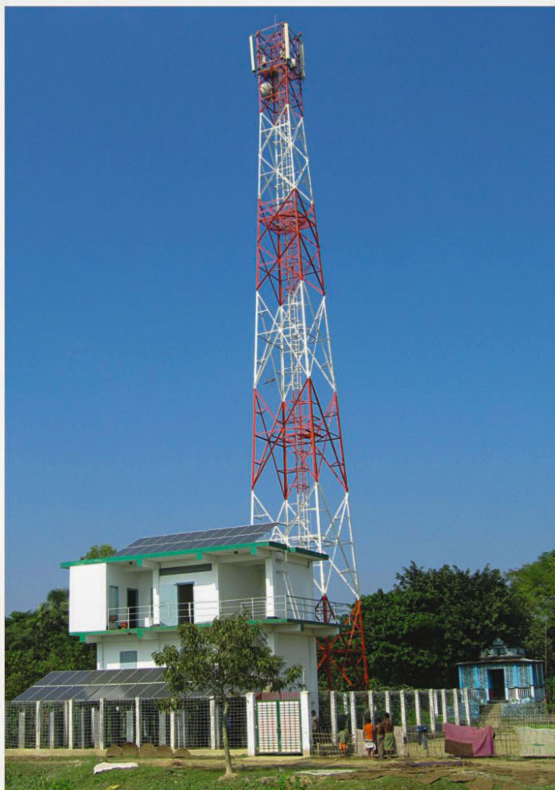
GRAMEEPHONE A base station of Grameenphone. Solar energy will replace diesel generators on 140 such sites of the leading mobile operator by the yearend.
