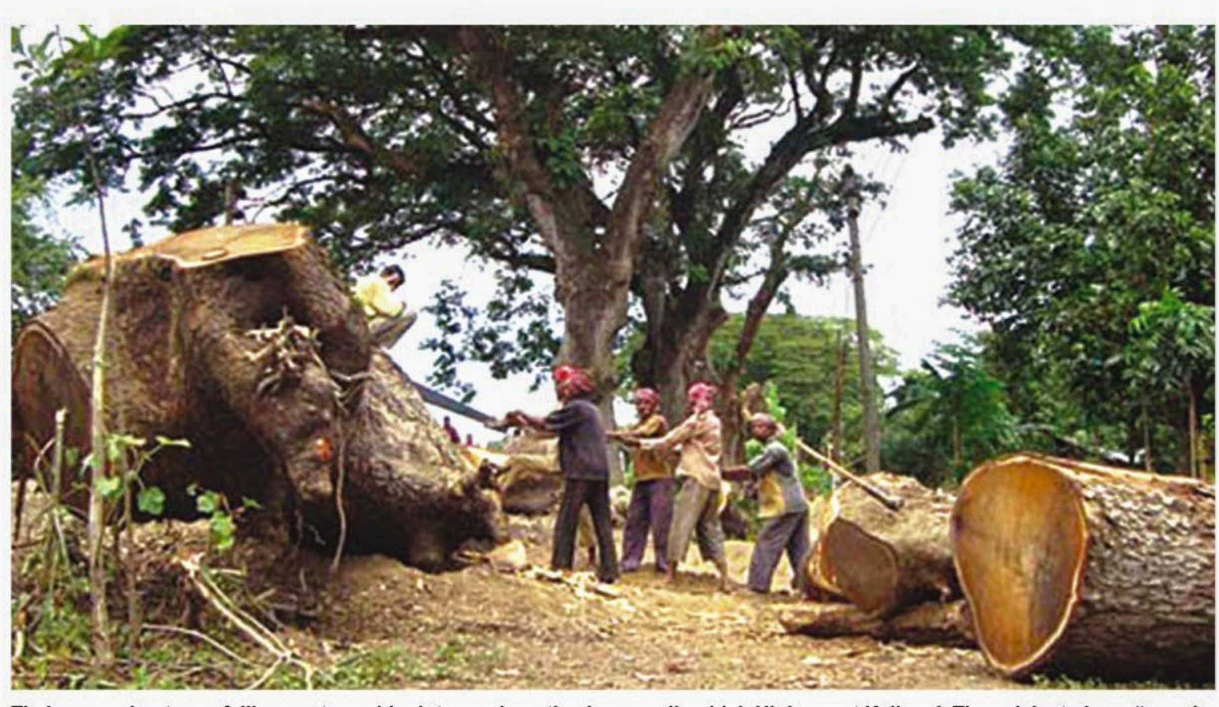
Timber merchants are felling century-old raintrees along the Jessore-Jhenidah Highway at Kaliganj. They claim to have "permission from Roads and Highways Department and a High Court order that clears their way for the plundering". The photo was taken on September 27 this year. PHOTO: STAR
