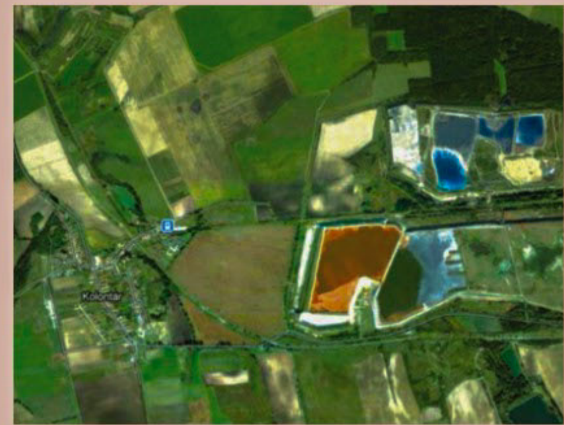
The bauxite residue holding pond (orange, middle), near Kolontar, Hungary (left), burst on Oct. 4, 2010
