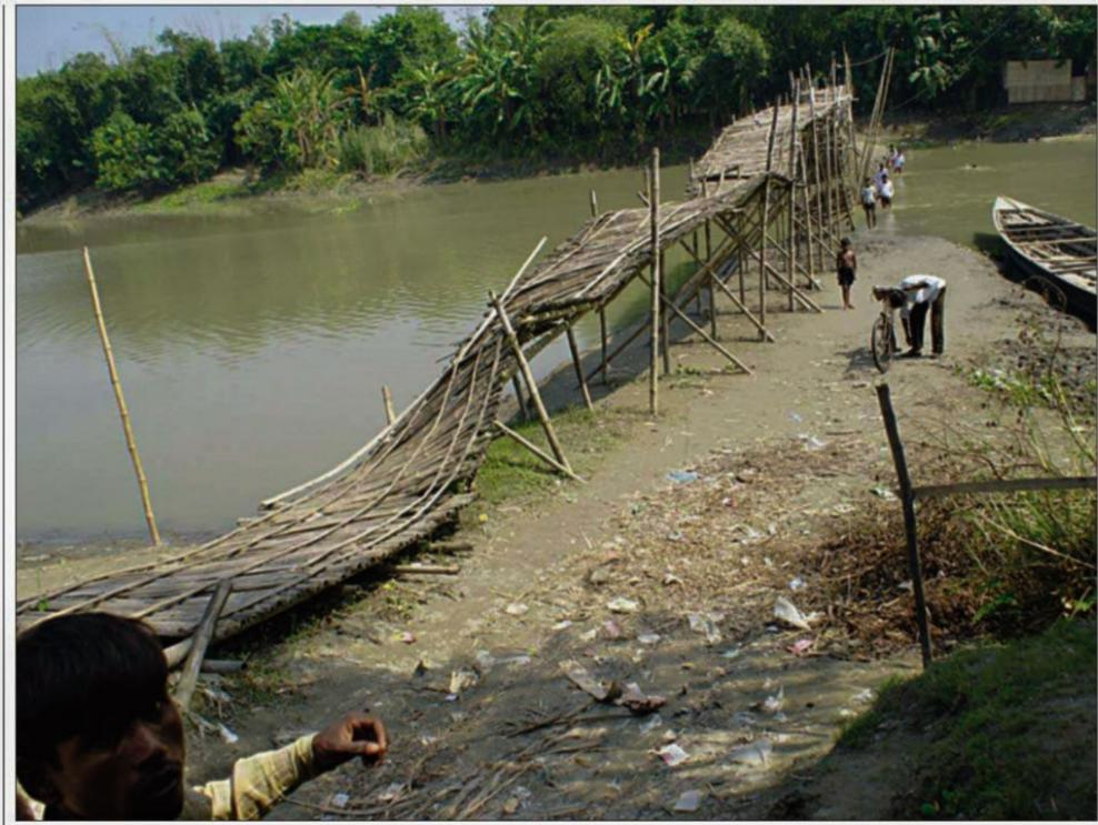
This bamboo-made bridge over River in Madarganj upazila of Jamalpur district collapsed recently, making construction of a concrete bridge all the more necessary to ease communication between Balijuri and Jurkhali unions and the upazila headquarters.
