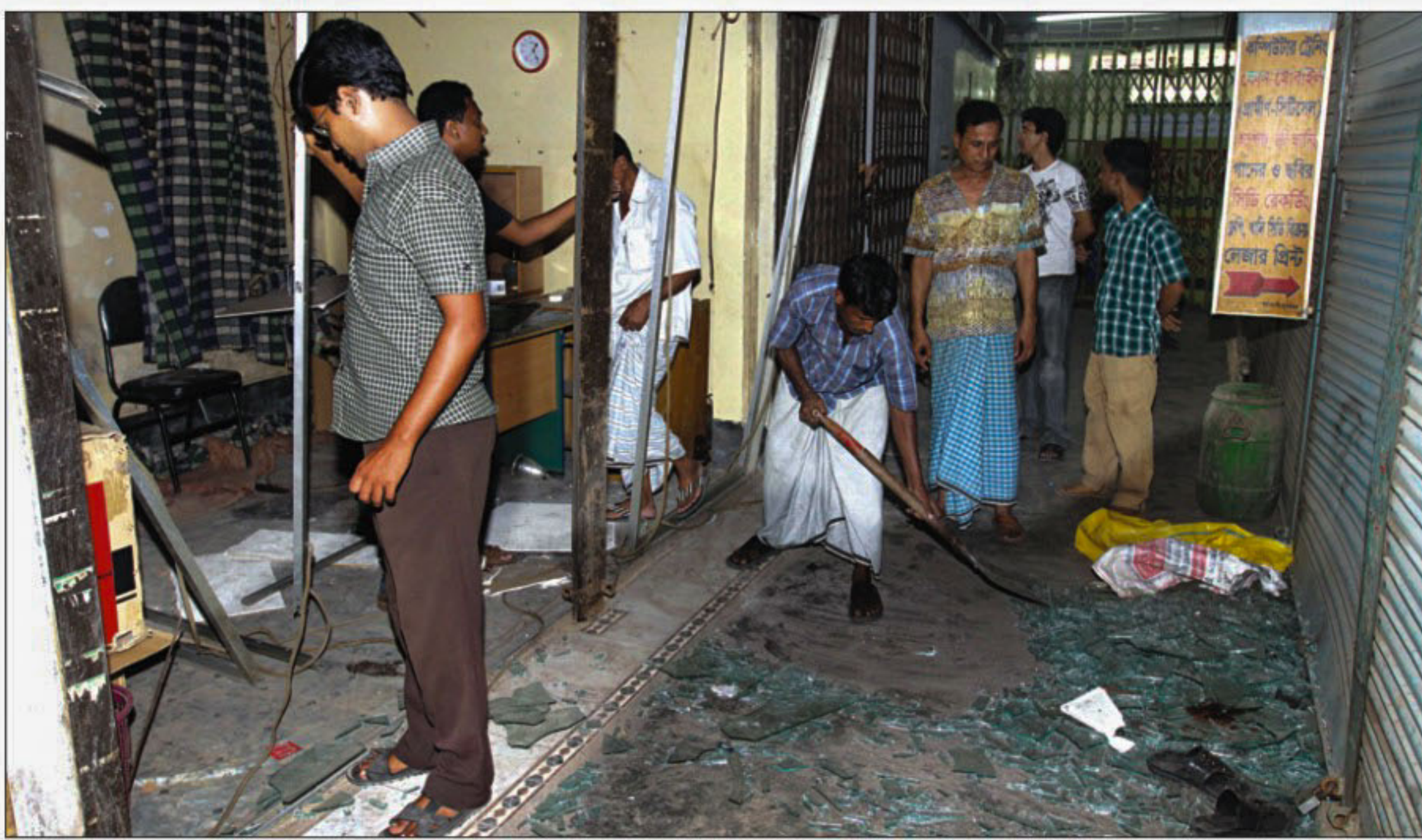
Glasses of a business establishment at Dholaiarpur in the city have been damaged as a safety tank inside it exploded yesterday.
