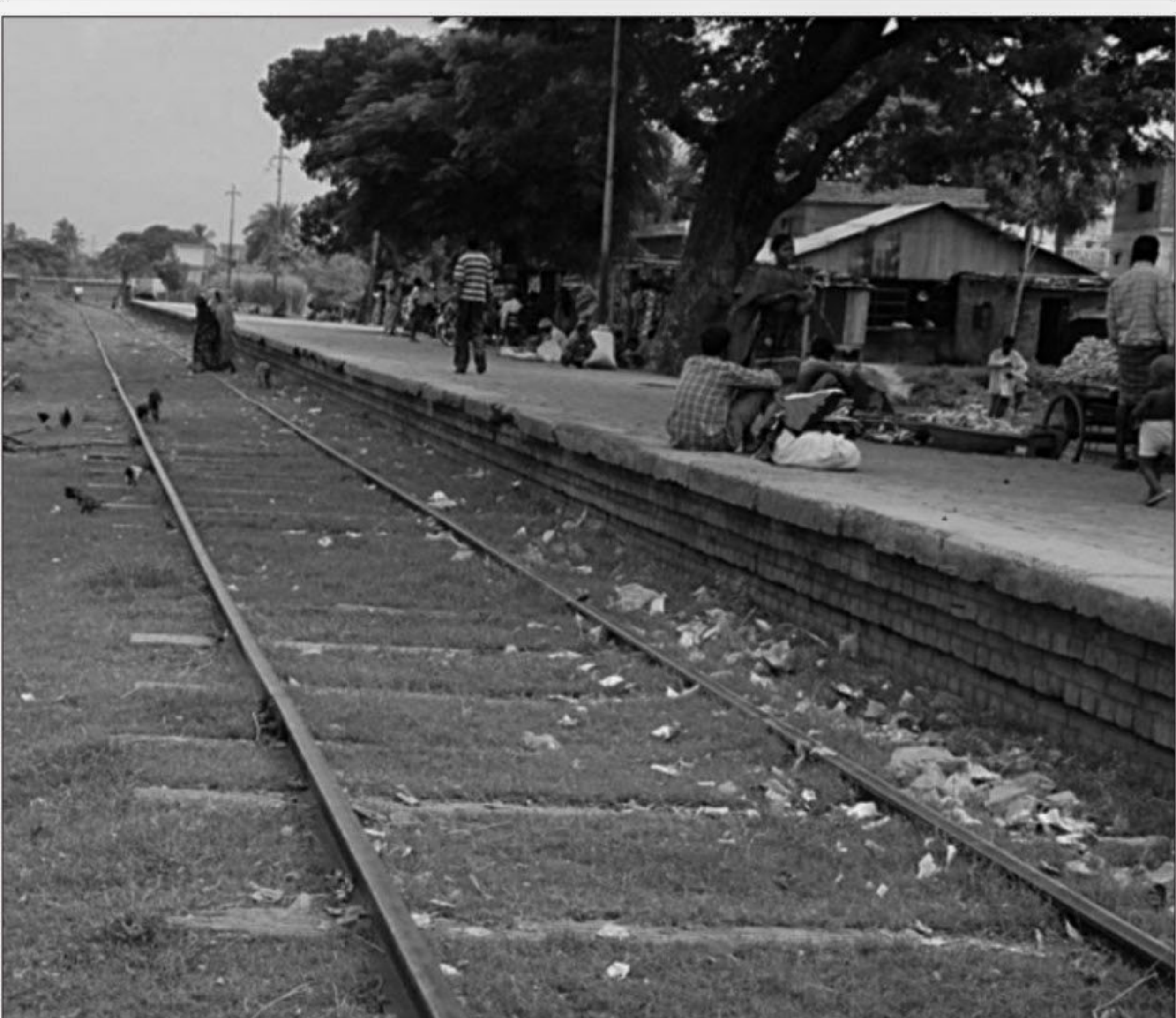
Railway tracks on Rajshahi-Chapainawabganj route have remained in an awfully dilapidated condition for long, causing frequent derailments despite very slow movement of trains. The photo was taken from near Rajshahi Court station yesterday.
