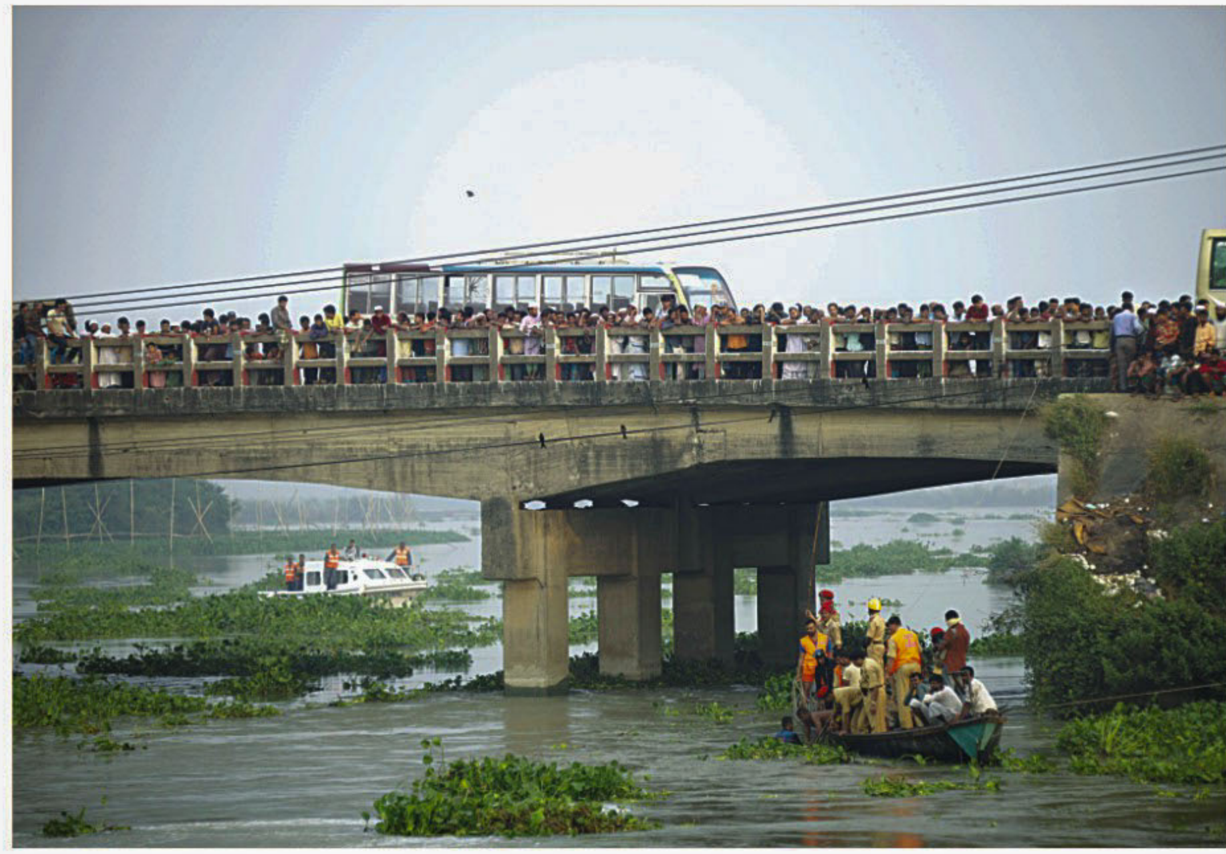
Salehpur bridge over the Turag river at Amin Bazar in Savar. Many people were killed in road accidents on and near the bridge in the last few years. On Sunday, a bus plunged into the river from the approach to the bridge, killing at least 13 persons. Experts say engineering flaws of the bridge are responsible for such accidents.
