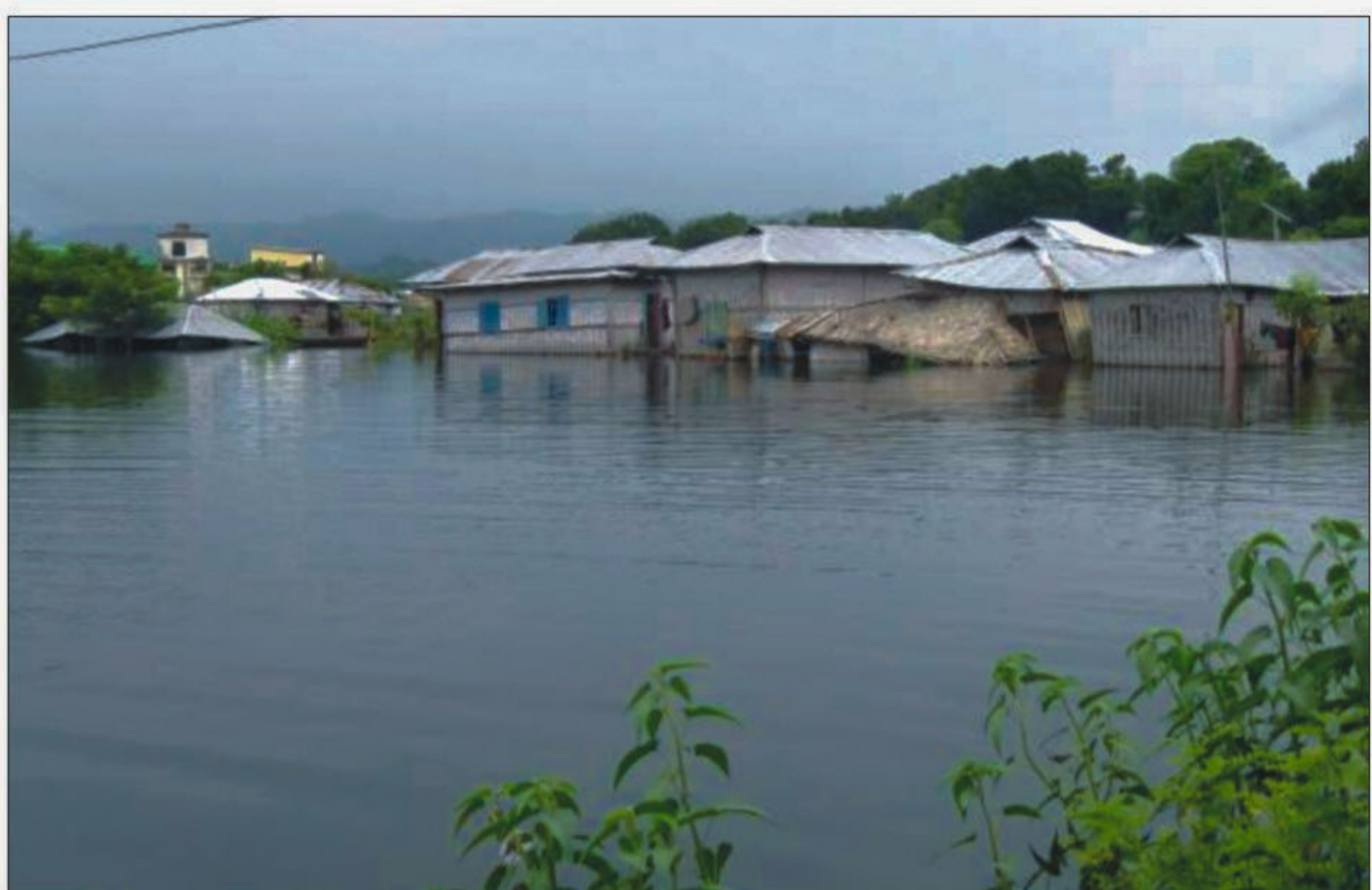
Fed by heavy downpour, overflowing Kaptai Lake floods houses at Kathaltali adjacent to Fisheryghat in Rangamati Sadar upazila.
