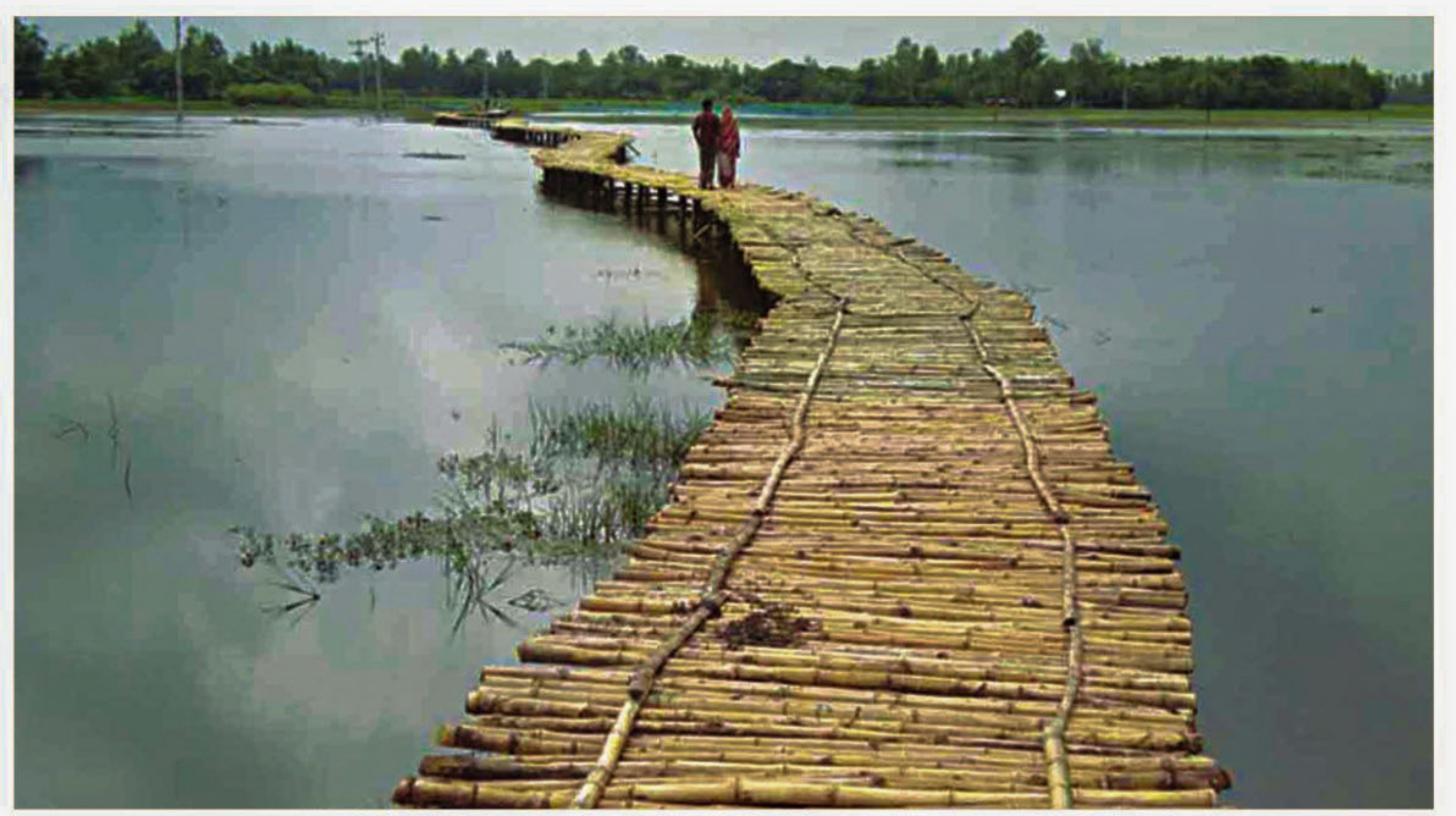
There used to be a road here. Subsidence due to coalmining underground claimed the only means of communication for the people of seven villages and left them with this primitive bamboo-bridge to negotiate. The photo was taken at Kalupara in Barapukuria, Dinajpur.
