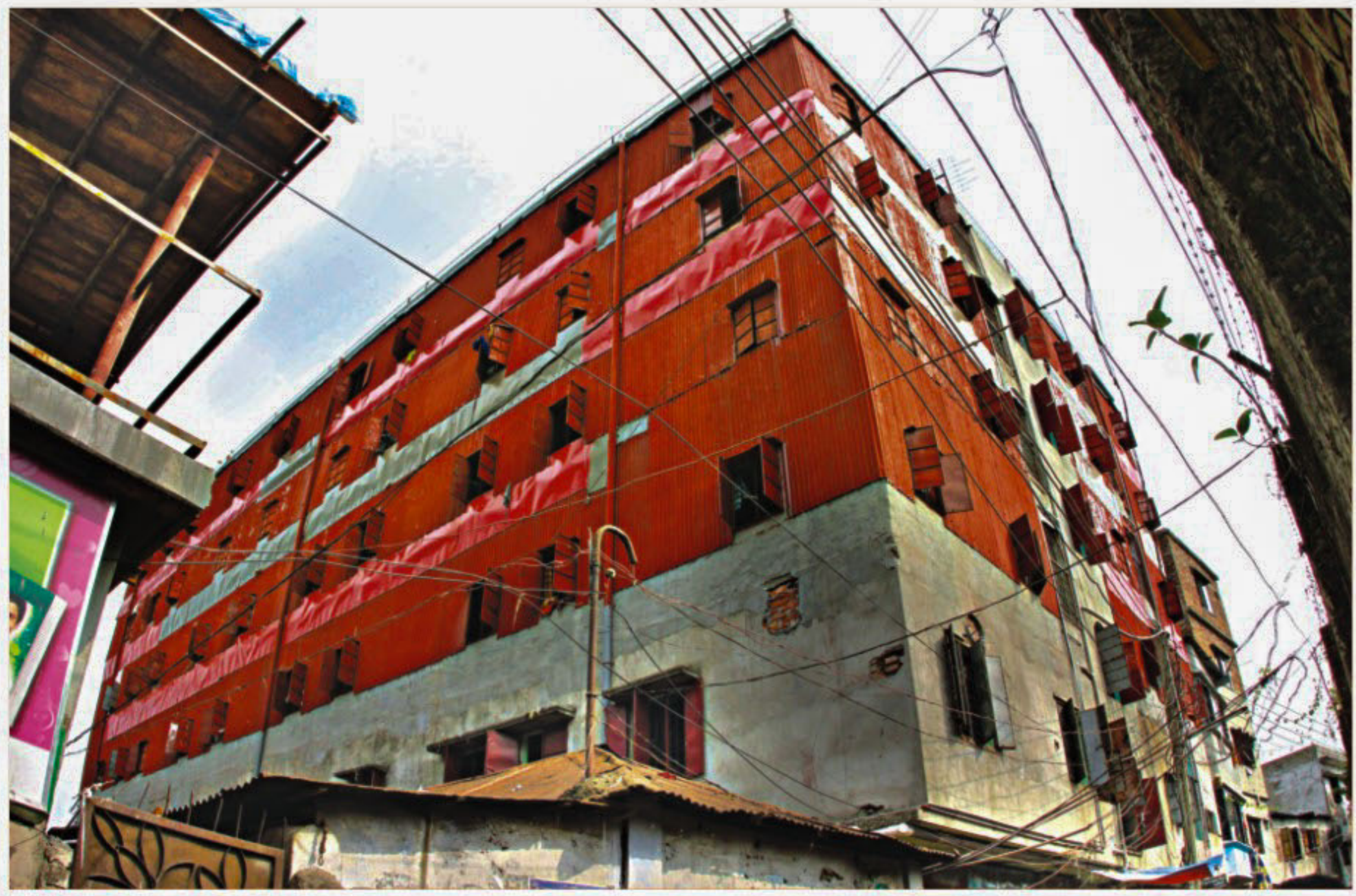
The building of toxic fume tragedy in Madhya Kunipara. The ground floor housed a dyeing factory while the top five floors "accommodated" around 1,200 people.
