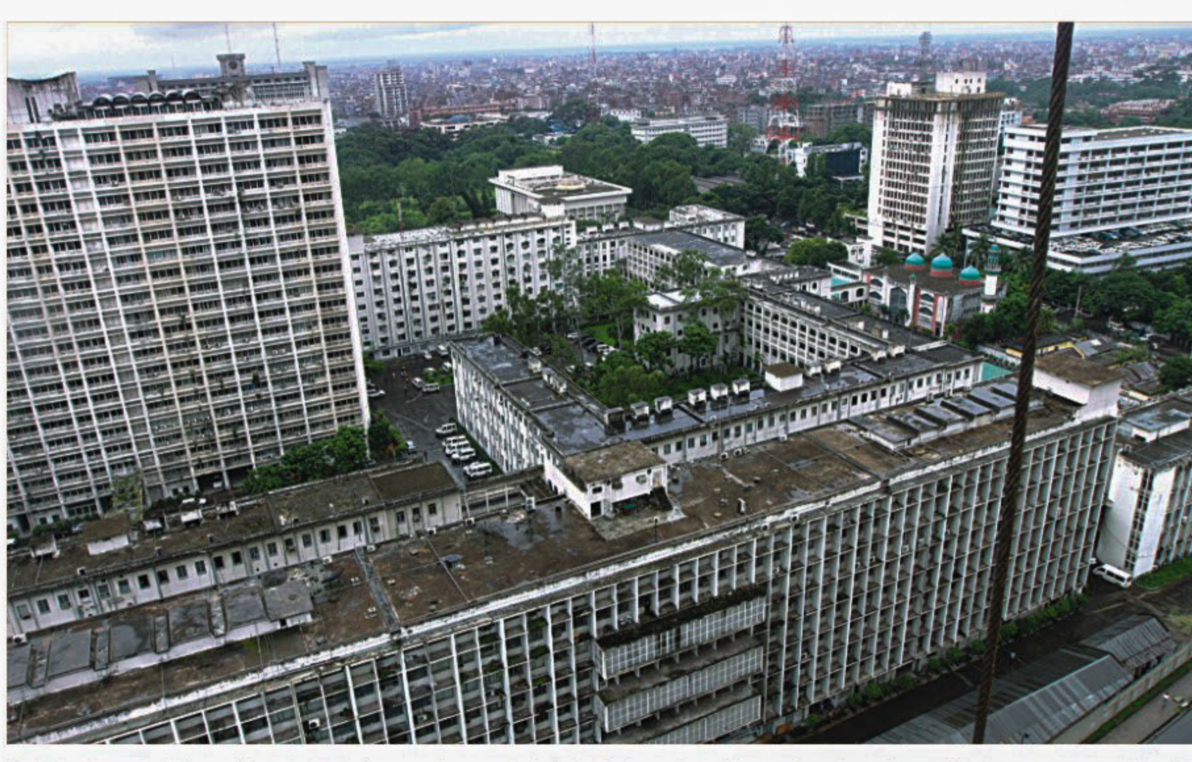
Only the large building of Bangladesh Secretariat, on the left, is designed to withstand earthquakes while the rest seven old buildings of the administrative hub remain vulnerable. PHOTO: SK ENAMUL HAQ
