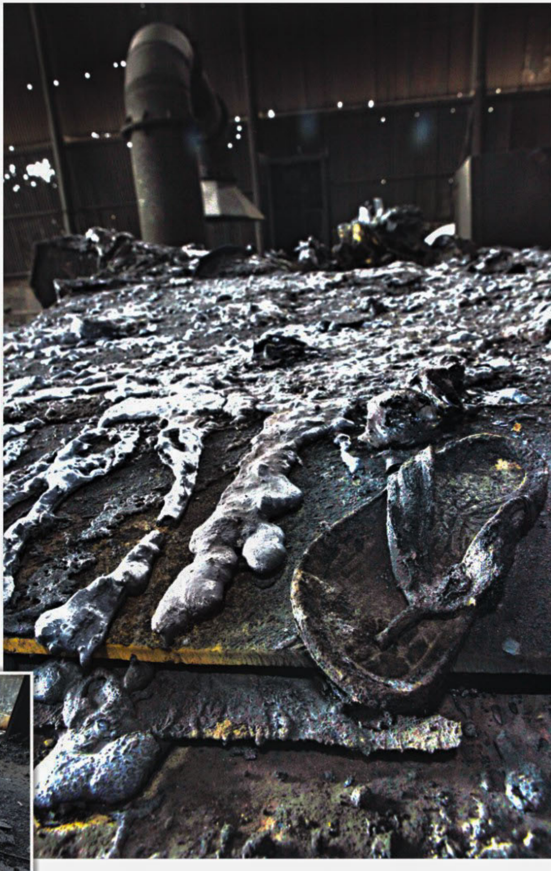
Left, A crater made by an explosion of a furnace at a steel factory. Top, Molten steel all around in the factory.
