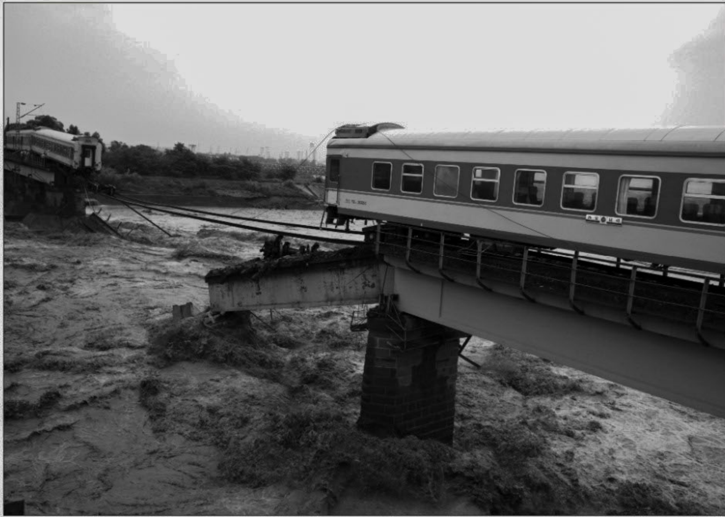
The two ends of a train remain on a bridge after passengers were evacuated near Guangan in southwest China's Sichuan province yesterday -- one of the areas hit hard by flooding that has plagued China in recent weeks. The train travelling in southwestern China derailed after floods destroyed a bridge, plunging at least two carriages into a river, but all passengers were safe.
