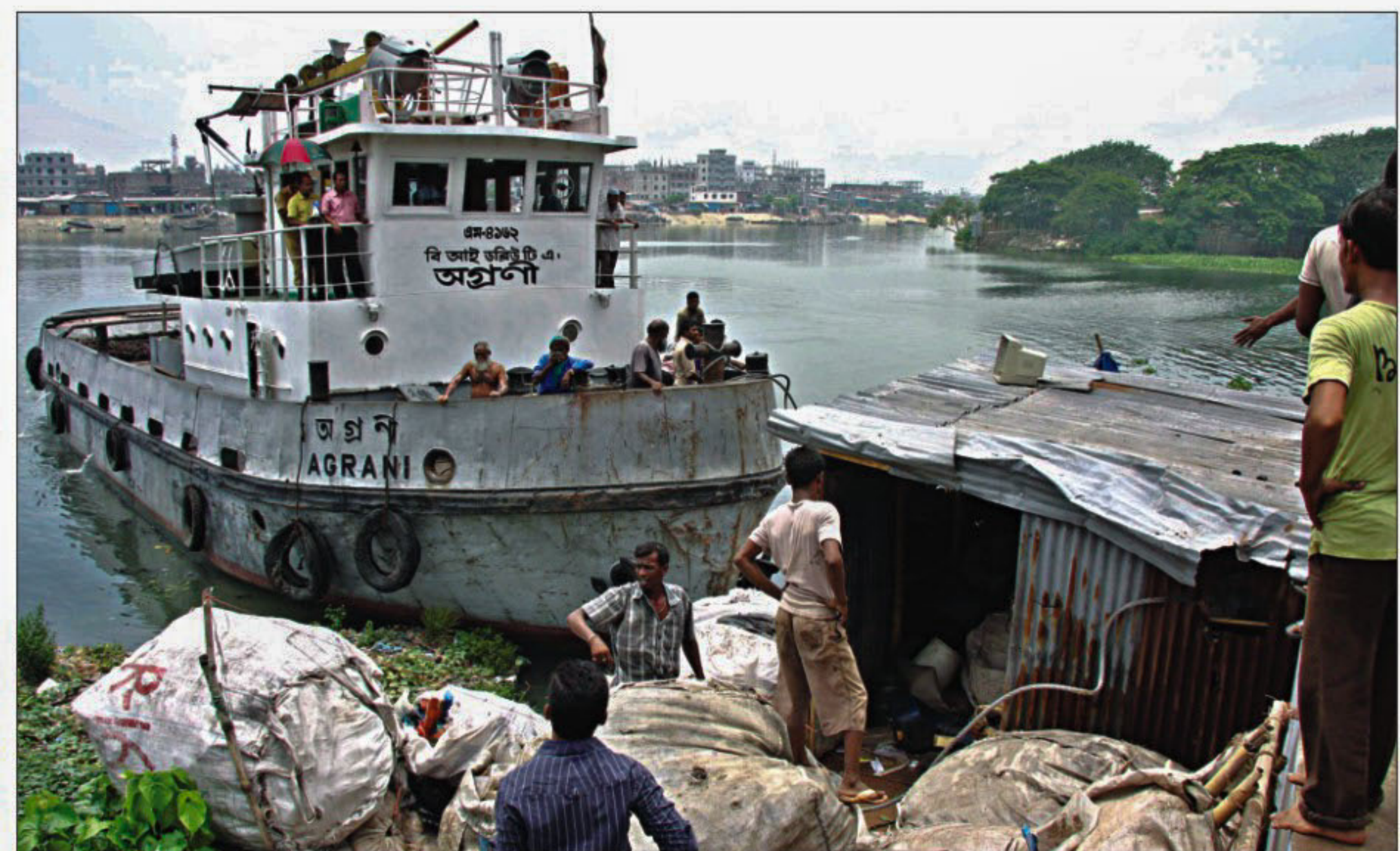
THE SHOW MUST GO ON!!! Bangladesh Inland Water Transport Authority (BIWTA) eviction team uses tugboat Agrani to knock down a tiny structure on the river Buriganga in Laibagh Beribadh area in the capital yesterday. The team was scheduled to demolish a salt factory encroaching 100 feet into the river but aborted the drive following law enforcers' refusal to arrange security force. Now it puts on the show of evicting a grabber.
