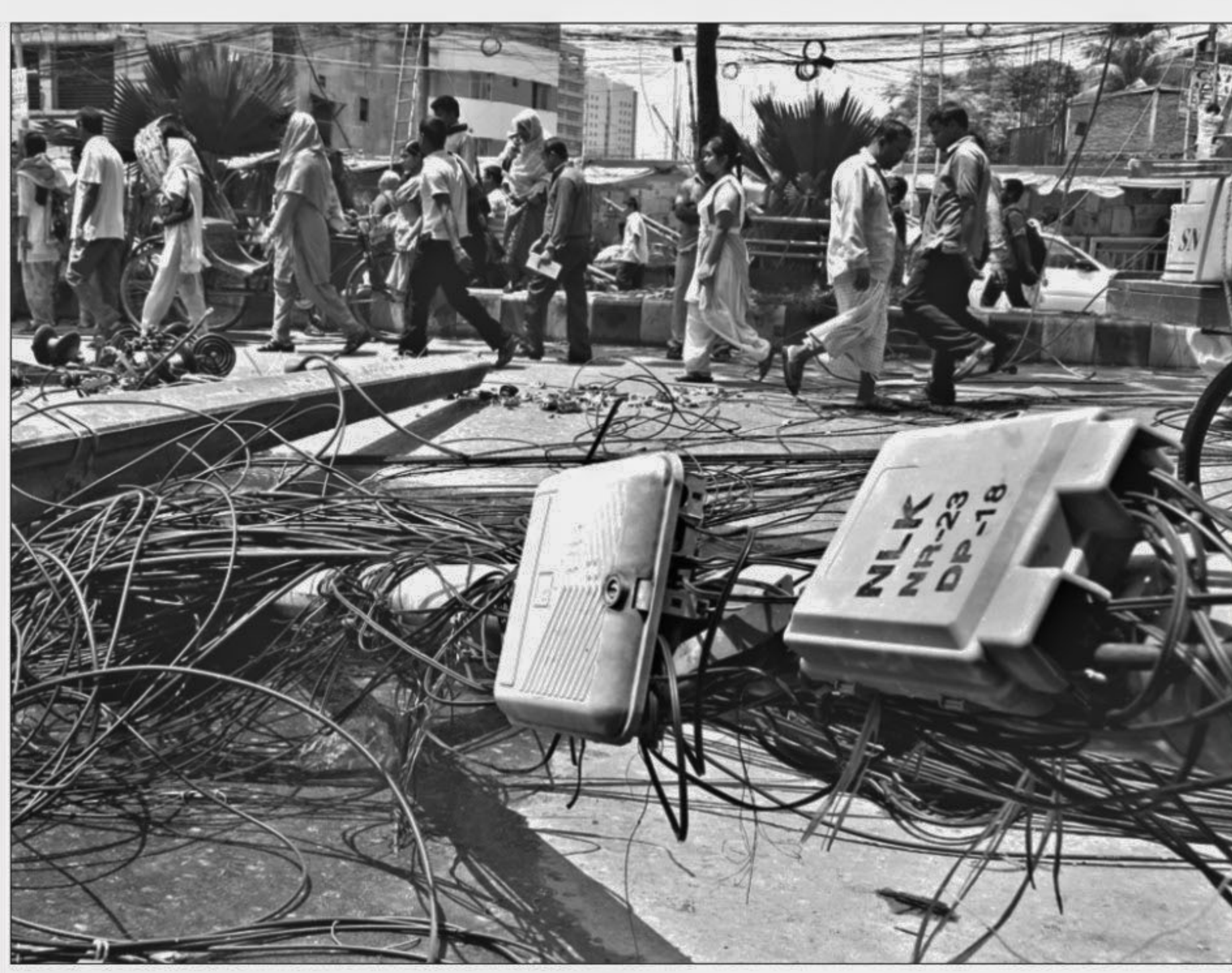
Electricity pillars brought down when a truck struck one of them and pulled down several of the serially connected poles between Bangla Motor and Shahbagh in the city disconnecting telephone, electricity and internet lines of the area yesterday.
