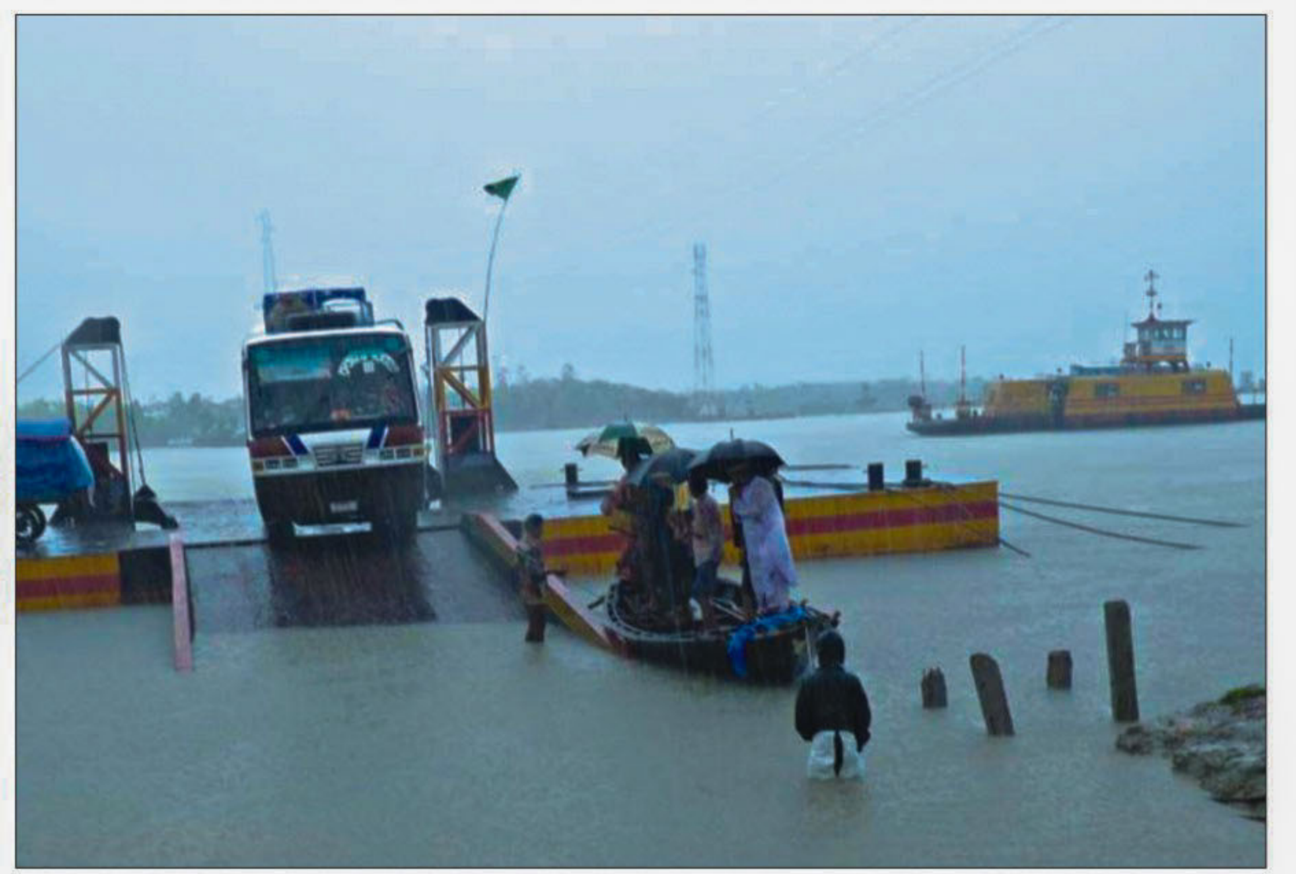
High tide floods the ramp and pontoon at Mohipur ferry terminal on Kuakata-Patuakhali Highway. A bus loaded with passengers is seen trying to get off the pontoon ignoring risks.
