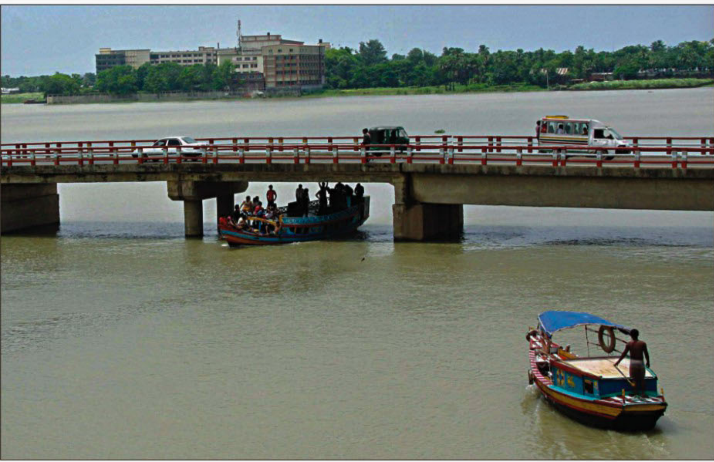
A boat sailing under this bridge on the river Turag at Ashulia almost touches the span over it. The bridge was built keeping so little space from the maximum water level that river traffic would be blocked if water level rises a bit more. The photo was taken a few days ago. PHOTO: SK ENAMUL HAQ
