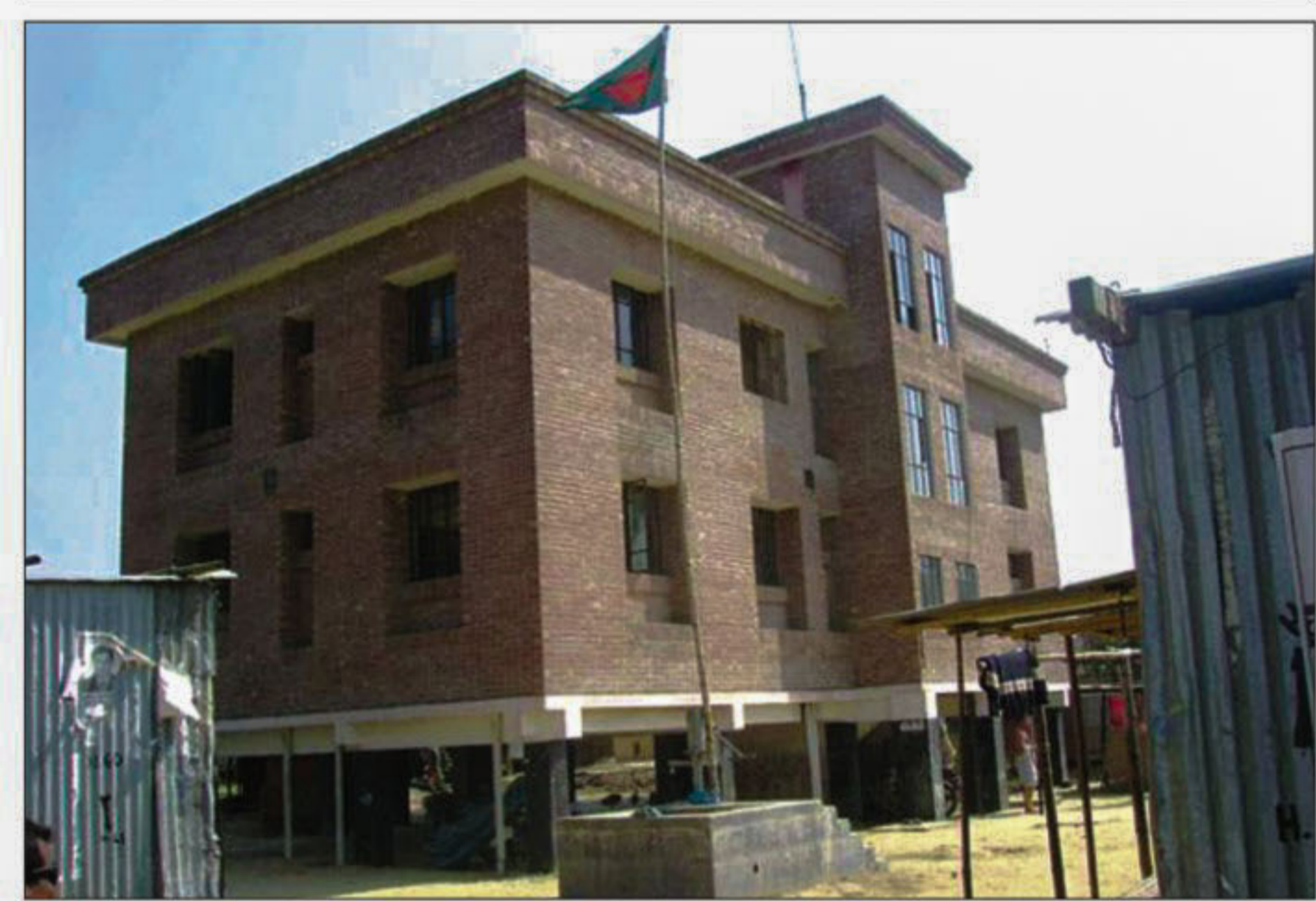
This health complex in remote Dhalarchar union in Bera upazila of Pabna district has been used as a 'temporary' police camp for the last three years, depriving locals of health services.
