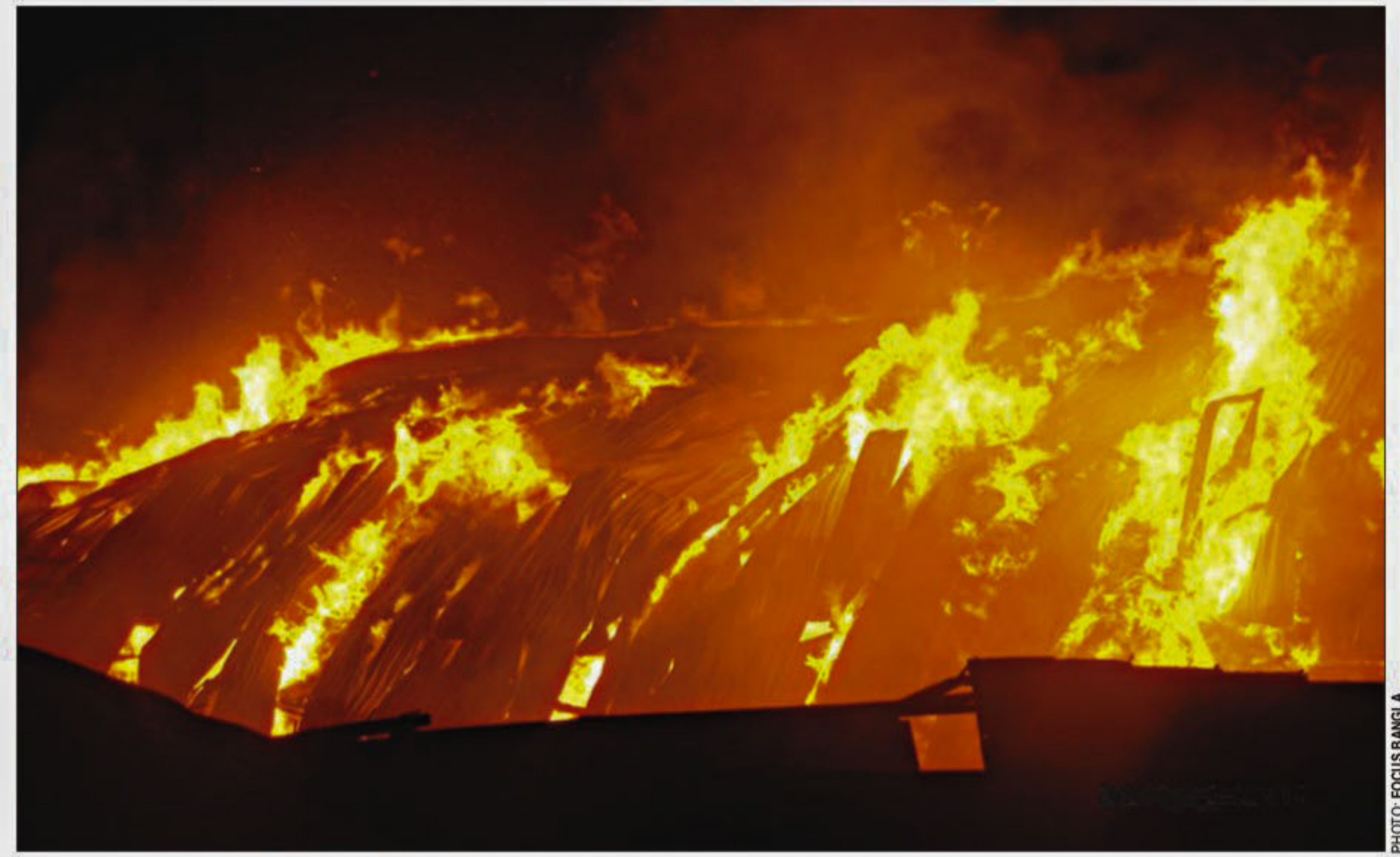
The raging fire at the Star Particle Board Mills Ltd at Narayanganj early today.
