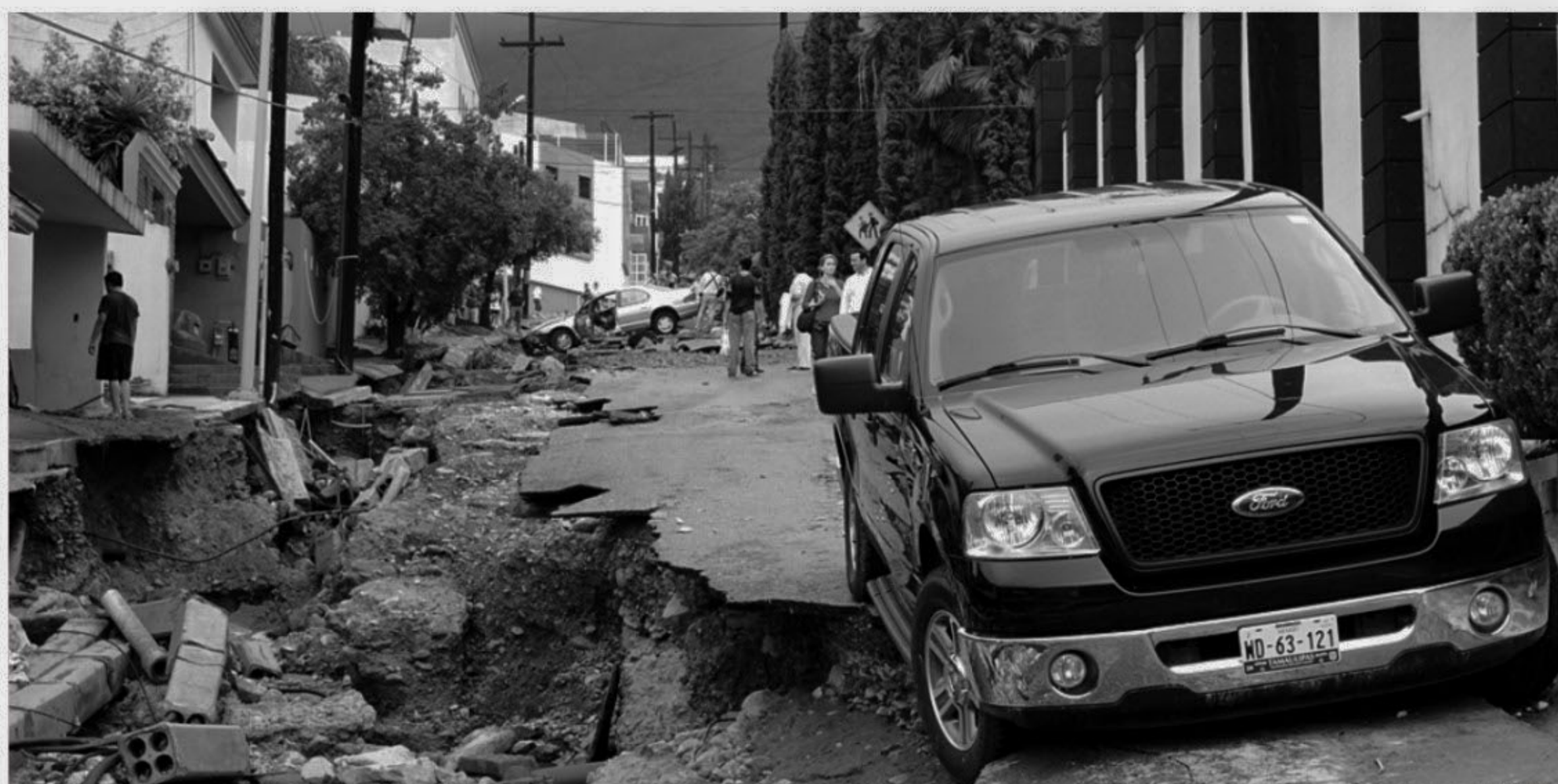
Overview of a sector heavily damaged by the overflowing of the Santa Catarina river, during heavy rains due to Hurricane Alex, in Monterrey, Nuevo Leon state, Mexico on Friday. Alex was downgraded to a tropical storm after roaring ashore late Wednesday as a Category Two hurricane slightly south of the eastern US-Mexico border.
