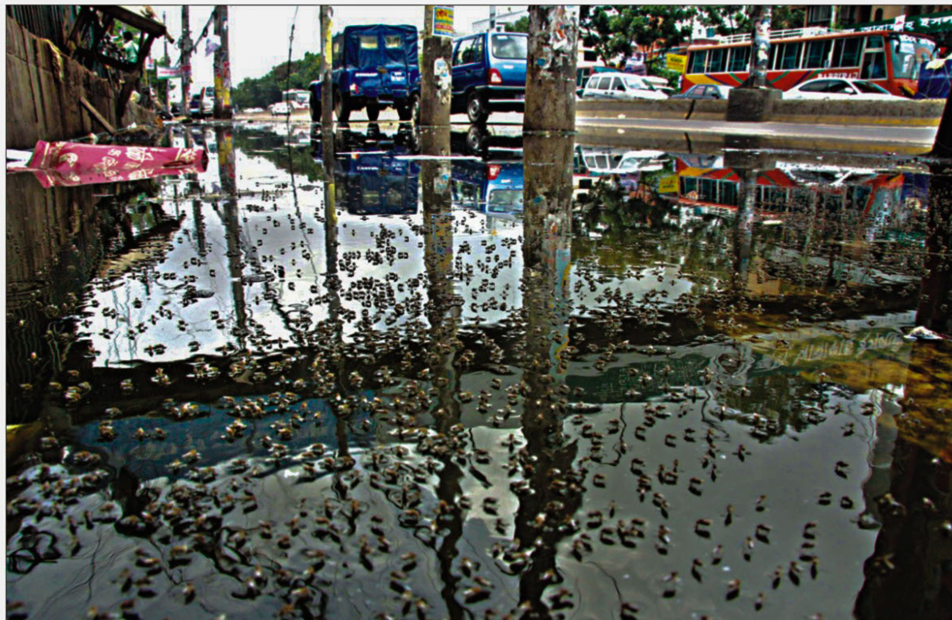
Due to poor drainage system, water remains stagnant on roadside near a footbridge at Uttara Sector No. 3 in the city, serving as a breeding ground for mosquitoes.
