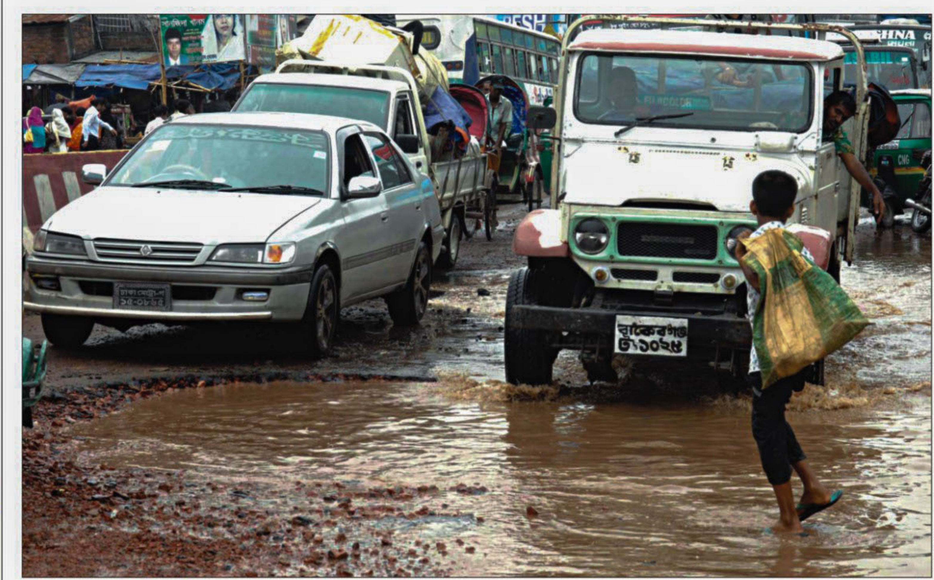
The condition of this road near Jurain Level Crossing in the capital has been in this sorry state for quite a long time, causing accidents frequently, locals said.
