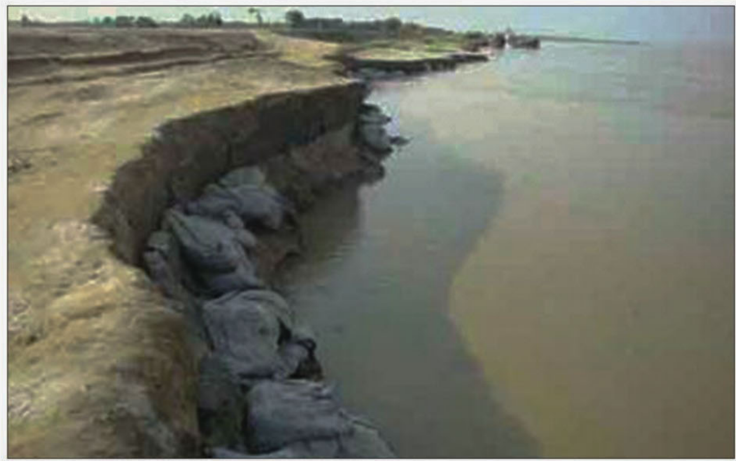
Water Development officials with the help of locals put sand bags in eroded portion to stop onslaught by the river Jamuna in Bera upazila. The site is only around 300 feet from Nagarbari terminal.
