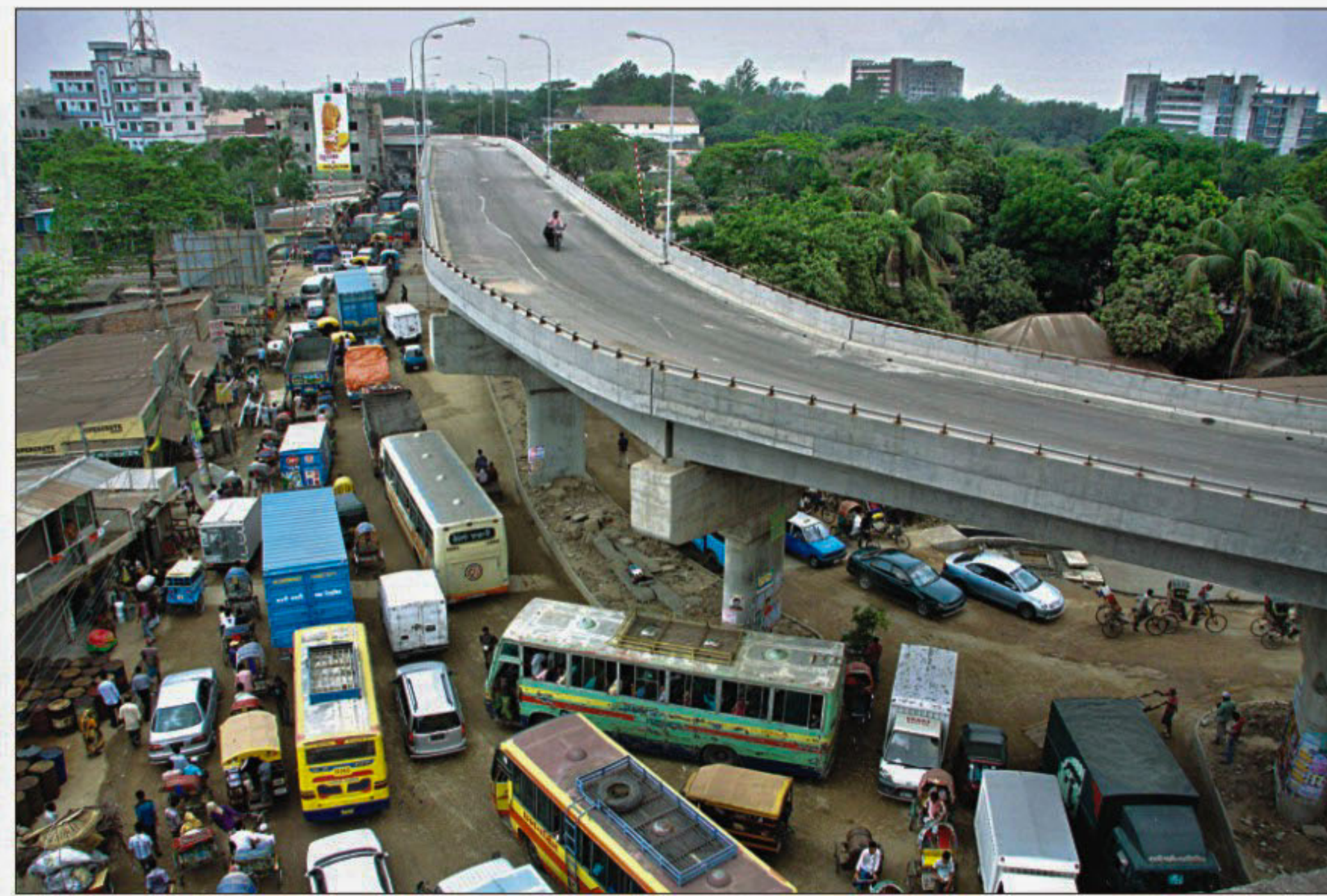
A section of the Tongi Overpass, which is soon to be inaugurated by the prime minister. The authorities missed the project deadline by two years due to a lack of proper planning, and faulty design. The delay also caused immense sufferings for local residents, and people who use the road. PHOTO: SK ENAMUL HAQ
