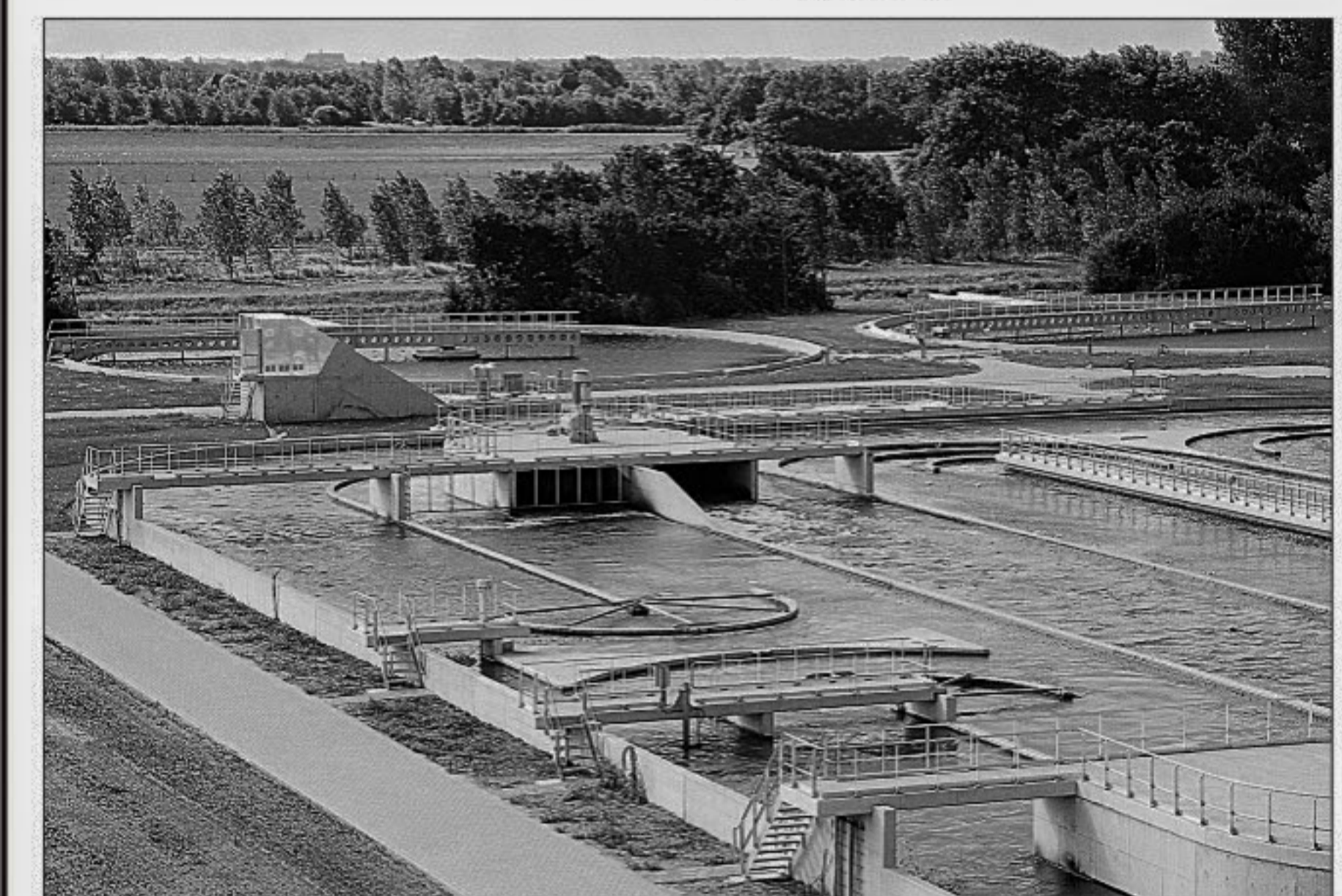
Biological wastewater treatment, Carrousel Geestmerambacht (Source: DHV)
