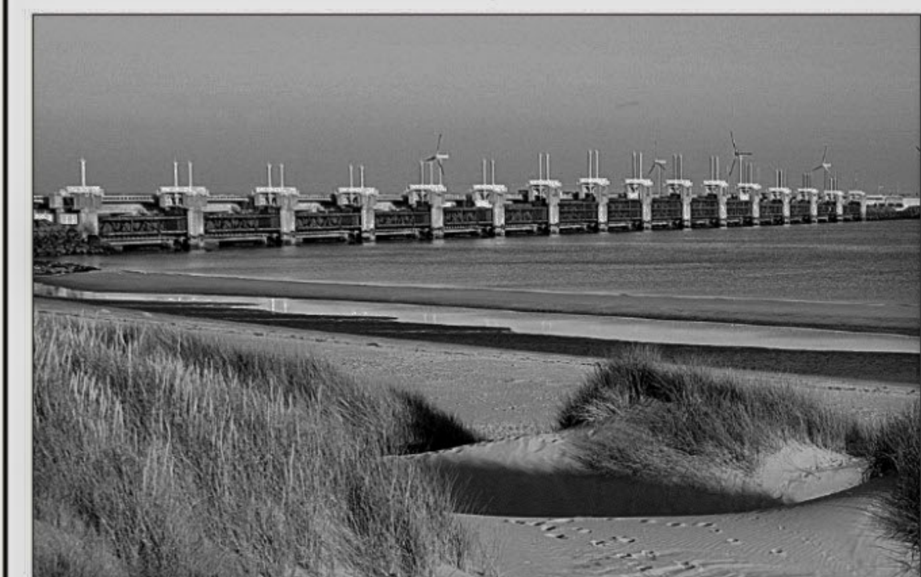
Eastern Scheldt storm surge barrier (Source: ©iStockphoto.com/Klaas Lingbeek-van Kranen)
