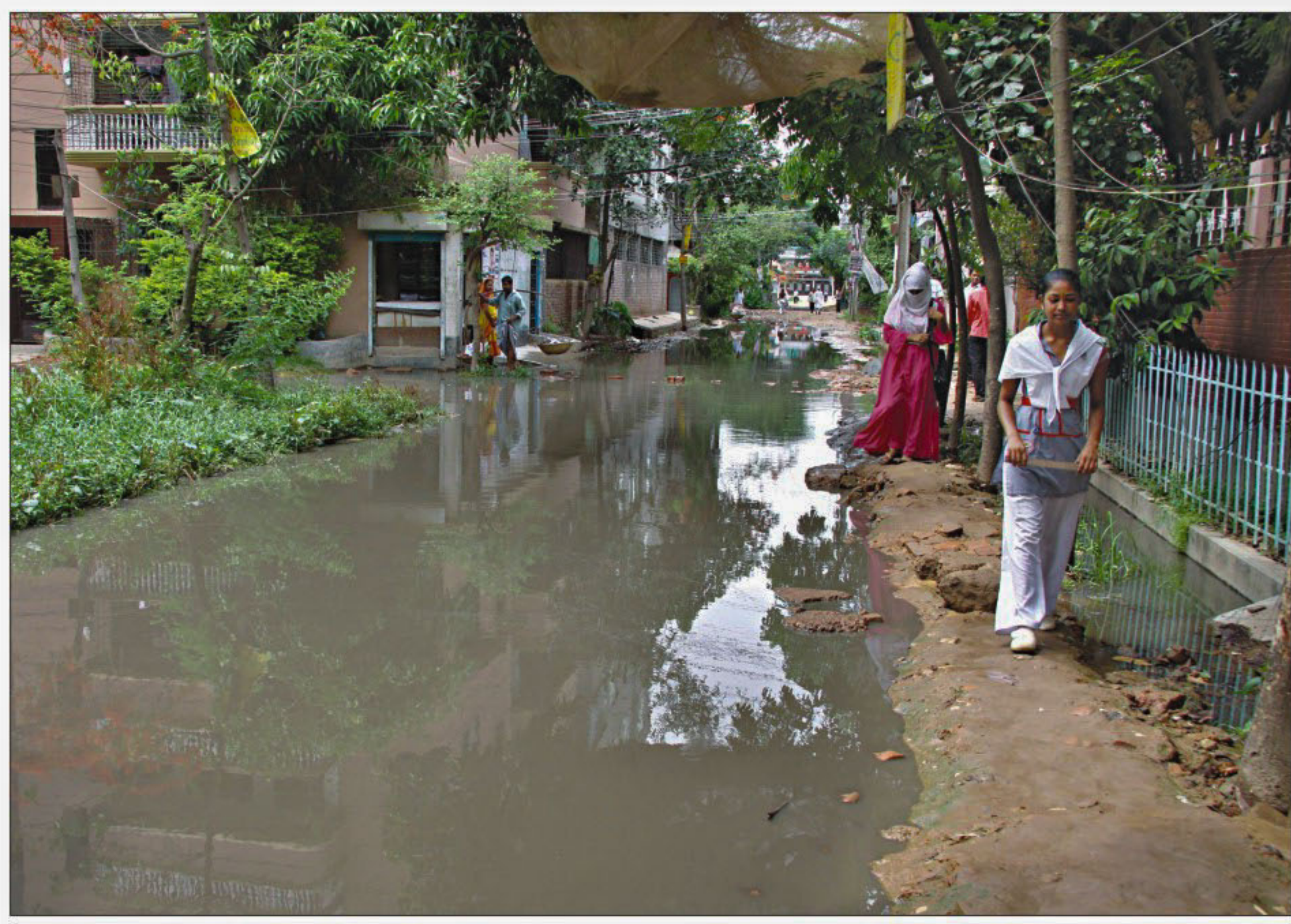
ROAD No. 3 at Nikunja at Uttara in the city remains under sewage water for long due to poor drainage system, causing immense suffering to road users, but the authorities remain indifferent to the problem. The photo was taken yesterday.
