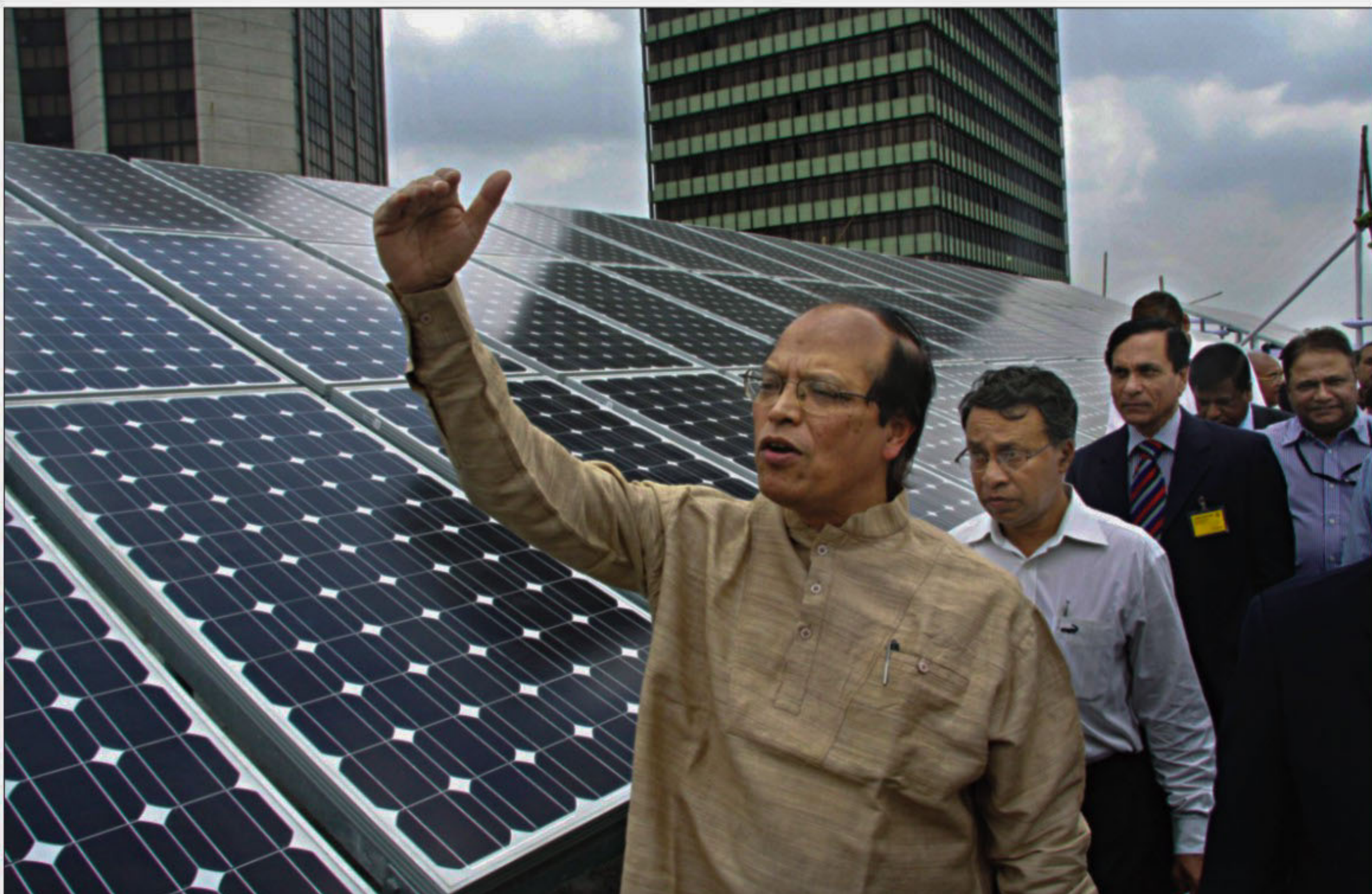
Atiur Rahman, governor of Bangladesh Bank, walks past an eight-kilowatt solar power system installed on the building's rooftop in Dhaka yesterday. Rahman described the move as indicative of the central bank's seriousness to increase power generation through renewable sources.
