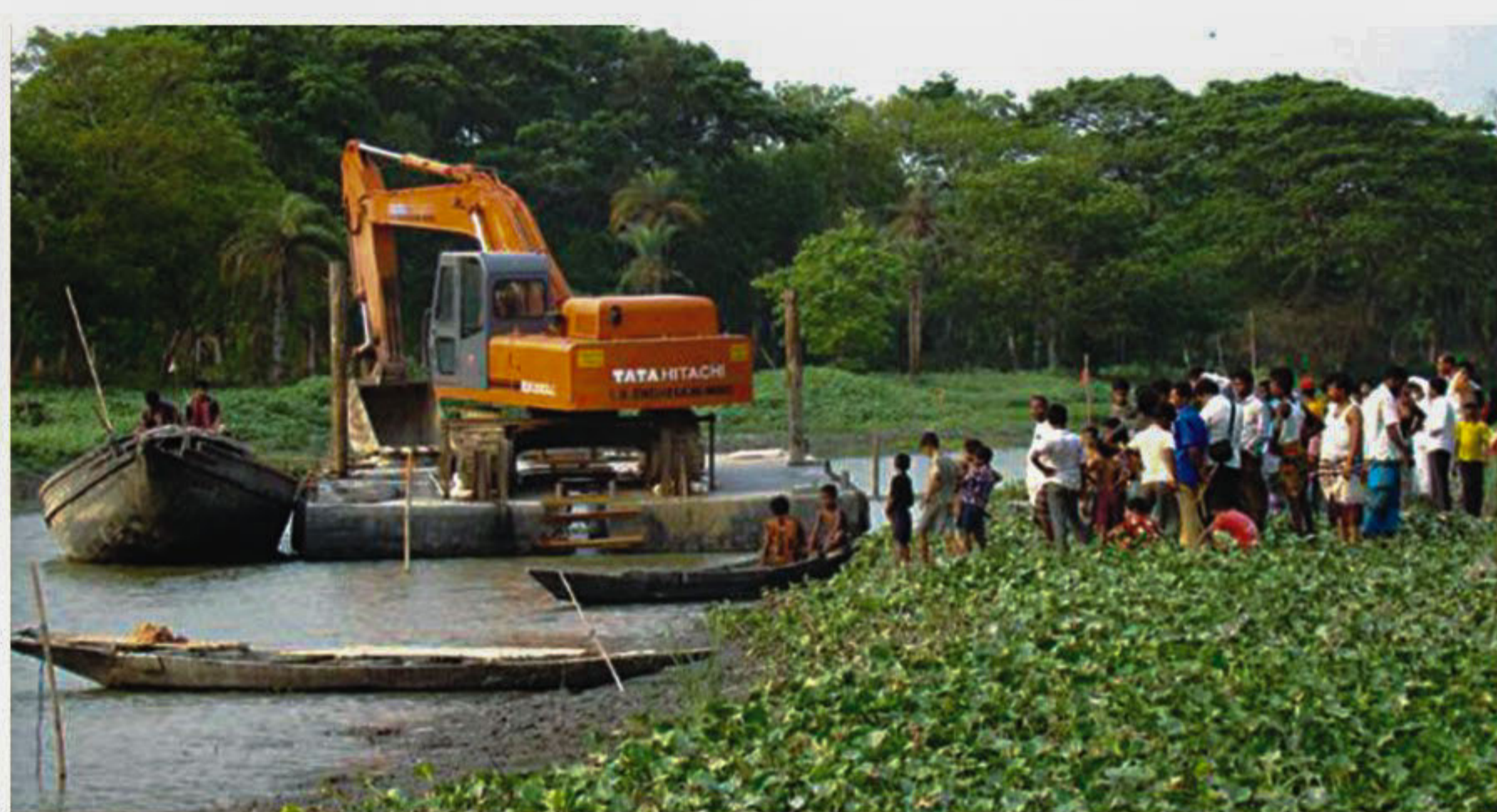
An Indian excavator on a barge removes silt of the Ichhamati at Pipili, West Bengal, India, while Bangladesh is yet to start dredging of the river. PHOTO: STAR
