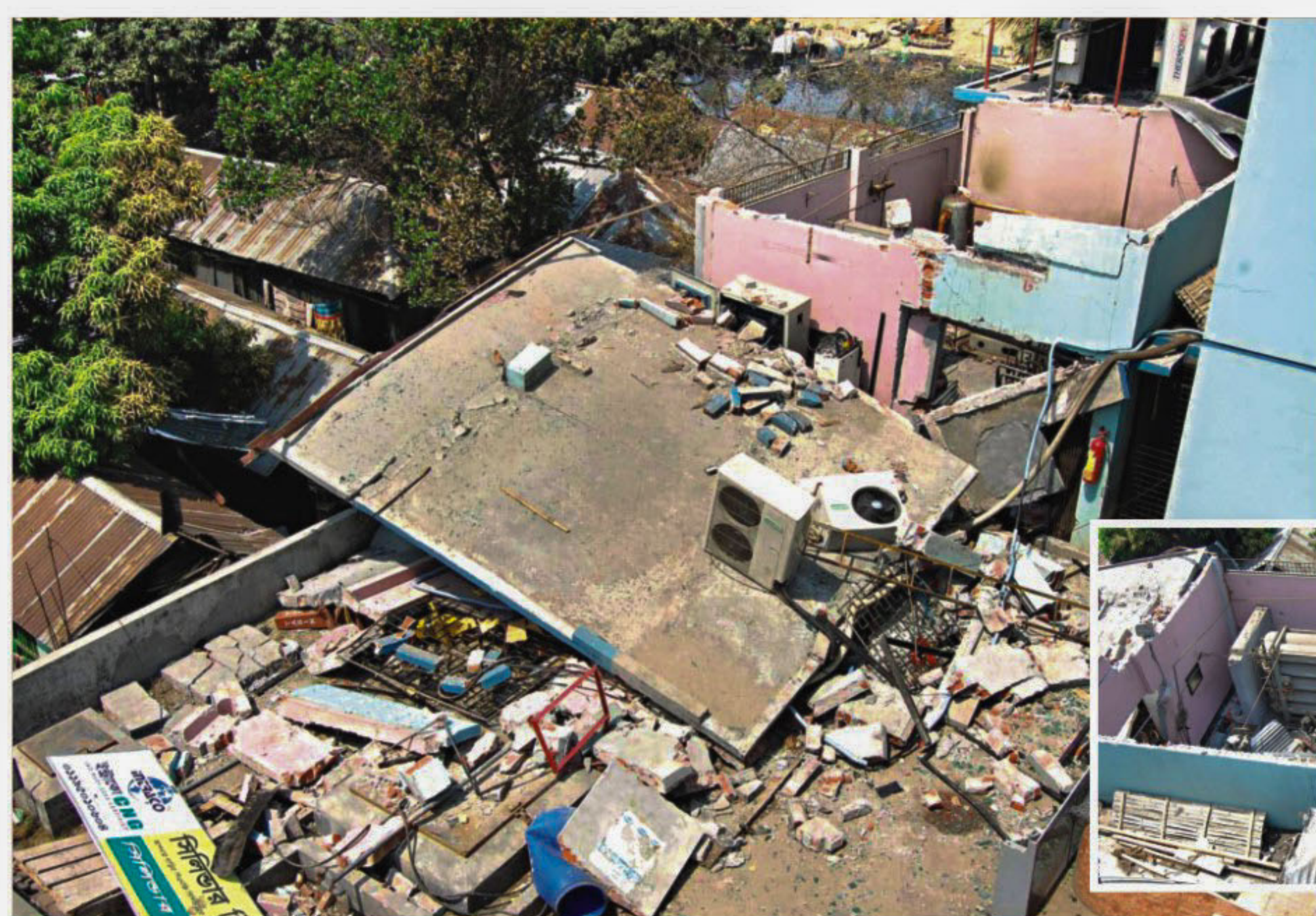
A huge explosion of the booster pipe at a CNG filling station in Uttara blew the roof of the station's electric control room on to a neighbouring building. The shock wave also damaged glass walls of the station's office nearby. Inset, the control room after the blast.
