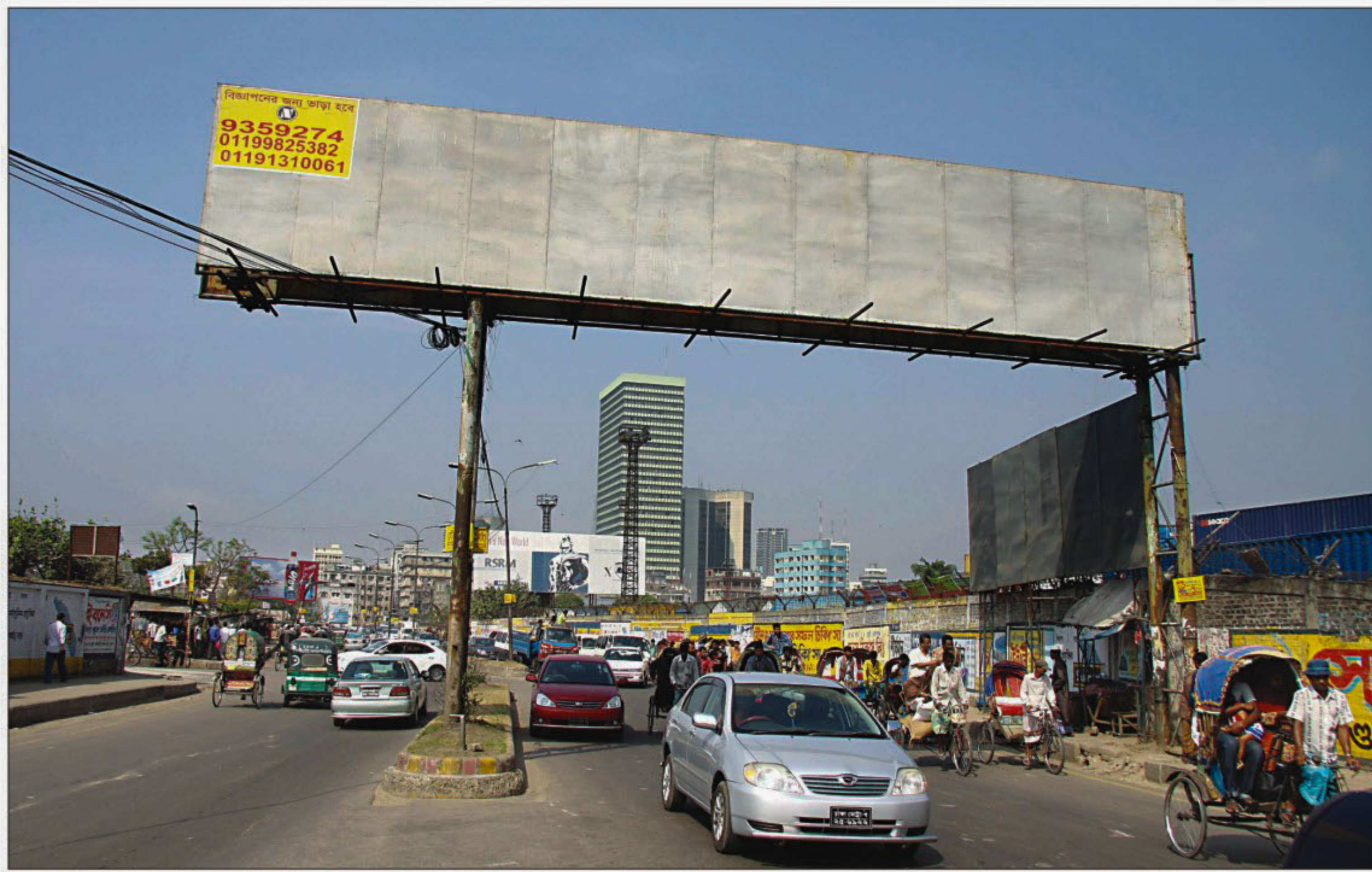
A hoarding built on a poor structure poses high risk of collapse especially in storm or strong wind. The photo was taken near the city's Kamalapur Container Station recently.
